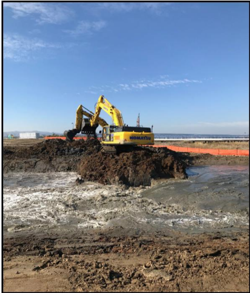
Breaching of levee at the Lower Walnut Creek Restoration Project, Martinez, CA Oct. 2021
