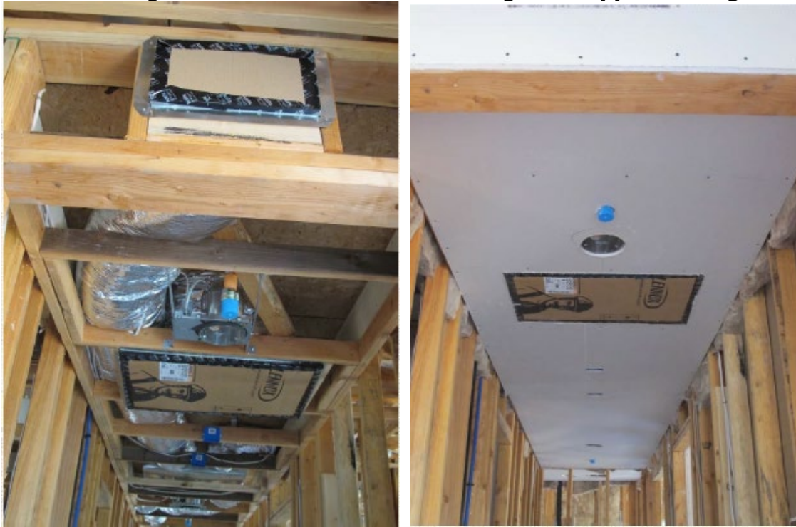
Figure 4-11: Ducts Routed Through a Dropped Ceiling
