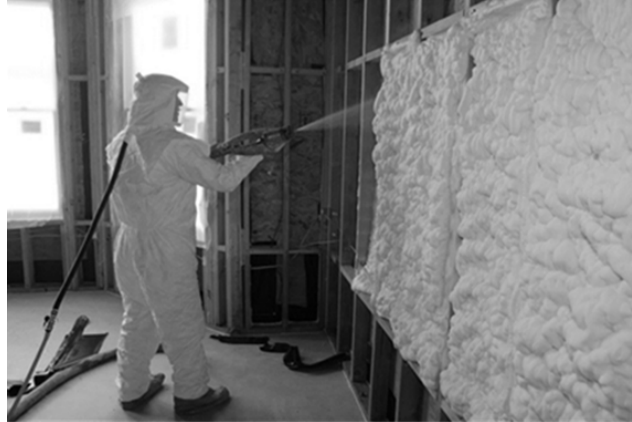
Figure 3-17: Open-Cell SPF Installed in Wall Cavity
