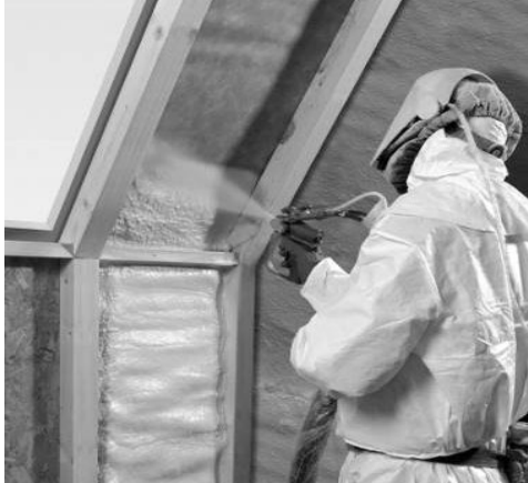
Figure 3-18: Closed-Cell SPF Installation in a Wall Cavity
