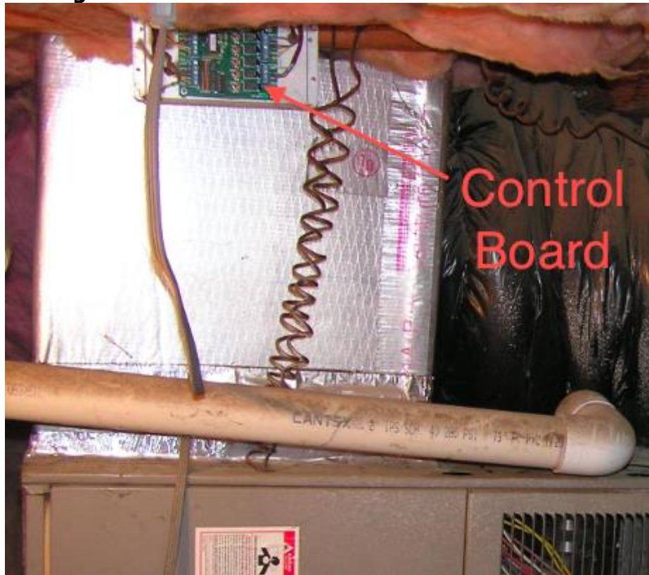
Figure 6: Photo of a duct-mounted control board.
