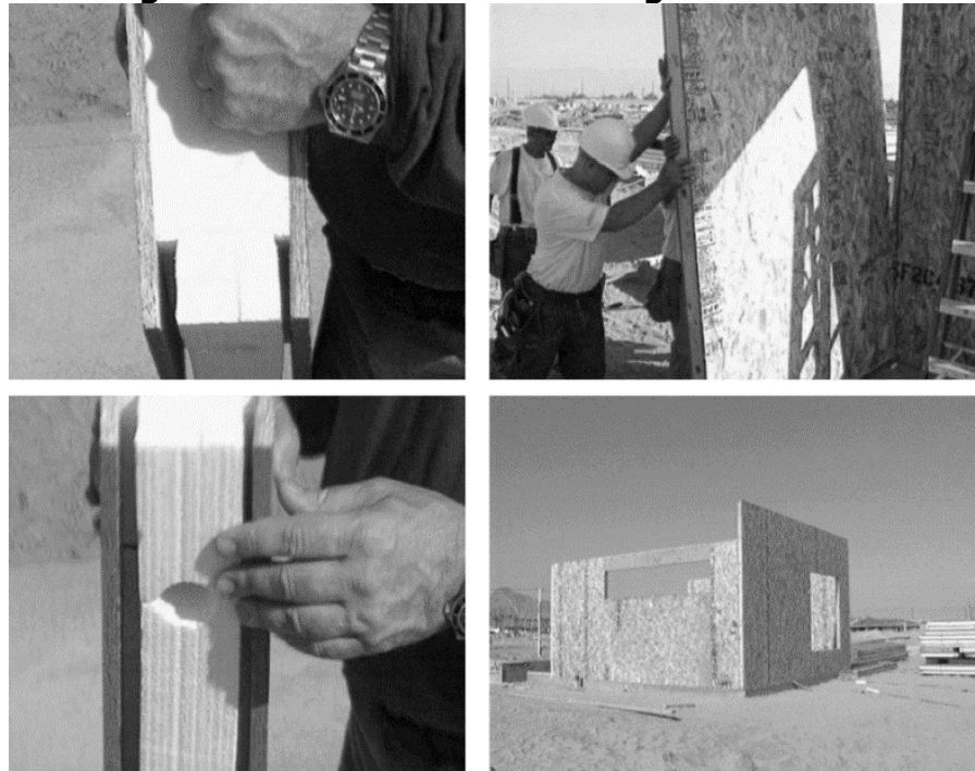
Figure 3-53: Methods of Joining SIPS Panels
