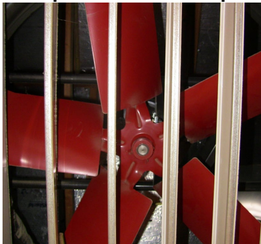
Figure 4-39: Open Barometric Damper With Fan Above
