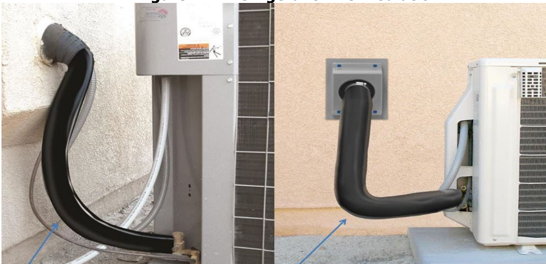
Figure 4-1: Refrigerant Line Insulation
