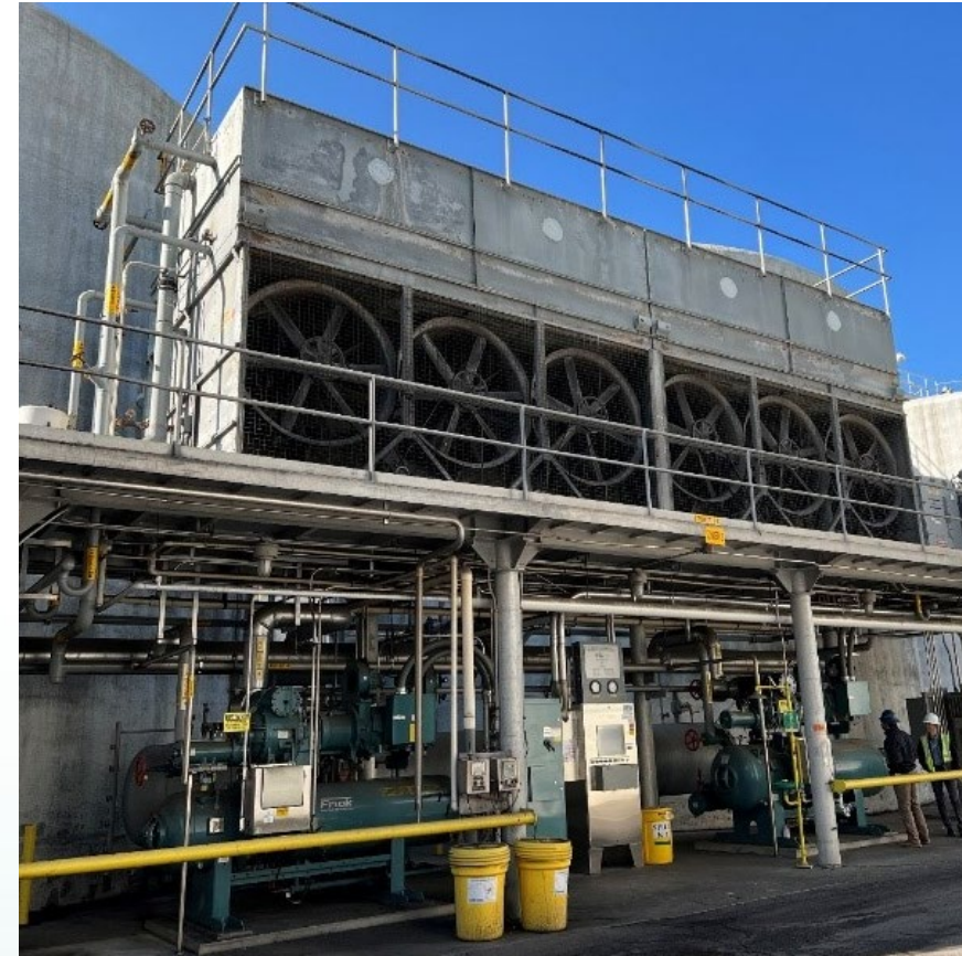
Outdated Baltimore air coil condenser at the Fresno's winery. Source: E&J Gallo Wineries
