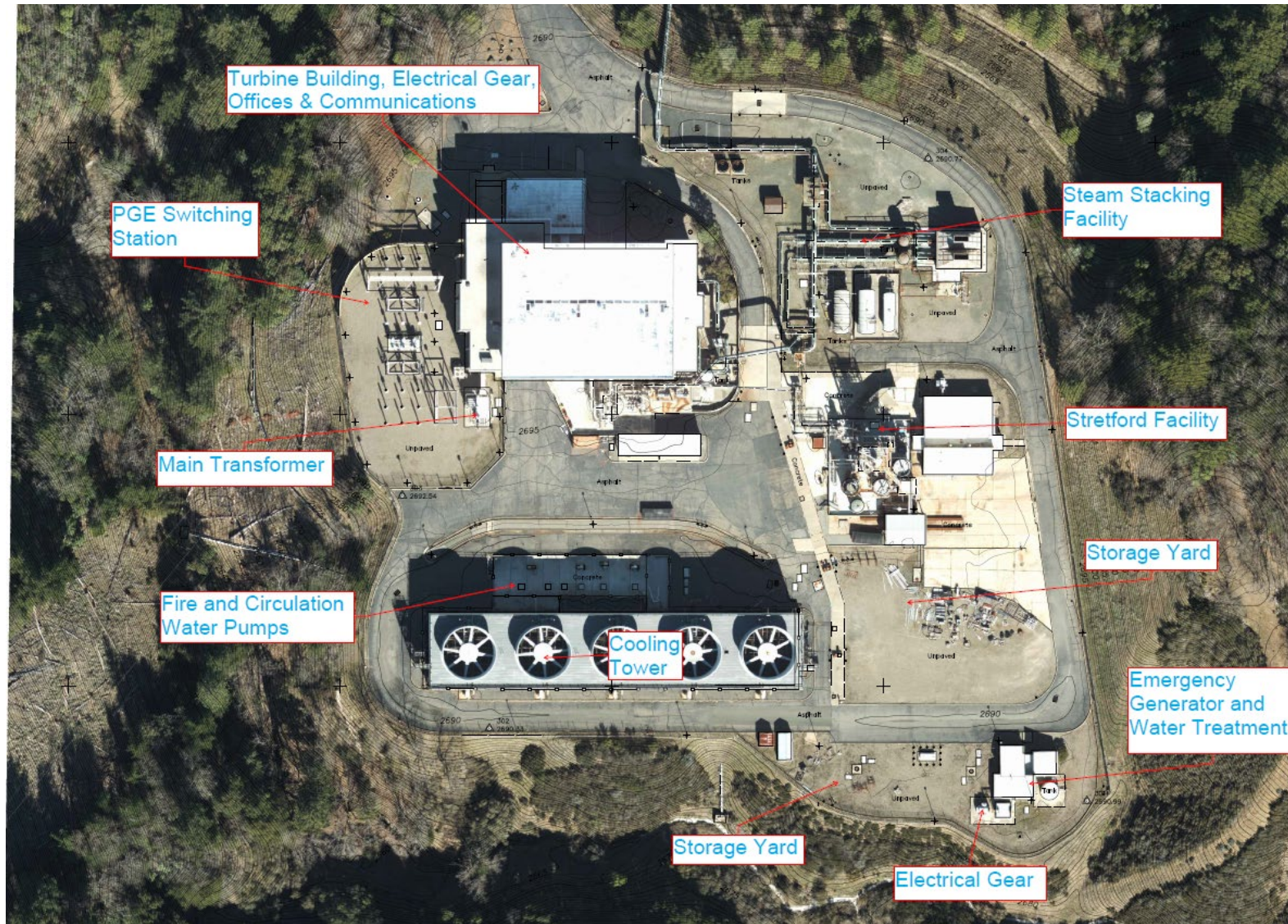
Figure 2.2-2 Existing Bottle Rock Power Plant Facilities
