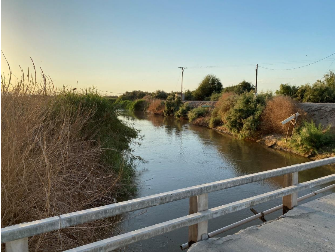
Figure 6-6. Overview of channelized Alamo River from Sinclair Road, facing northwest.
