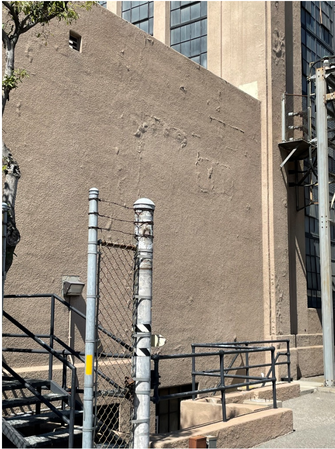
Photograph 3: Station A, southeast corner, facing northwest.
