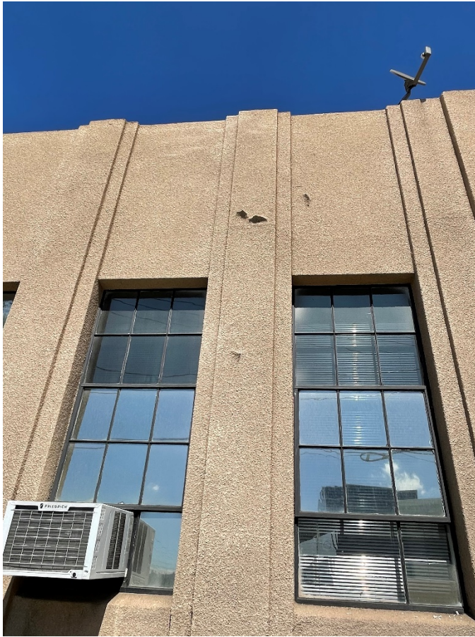
Photograph 6: Station A, ground floor, facing north.
