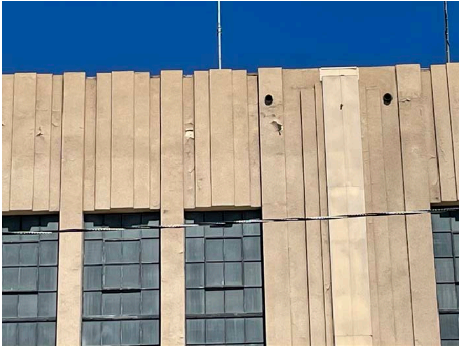
Photograph 5: Station A, upper floor, facing north.
