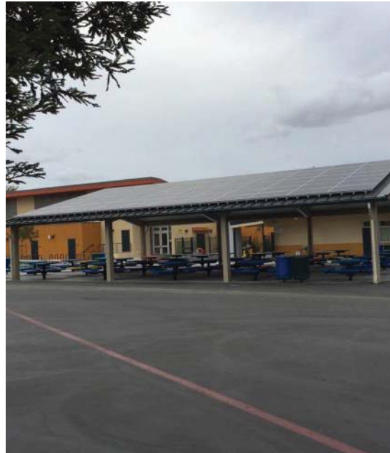
Solar Lunch Shelter at Lynhaven School
