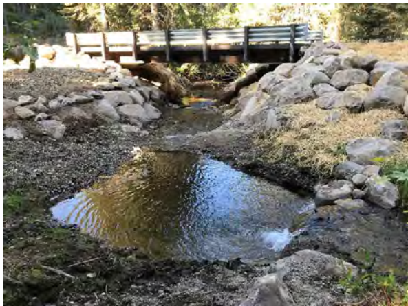
Photo 26. Cedar Creek, a perennial stream (data points 42-44). Adjacent riparian wetlands are recovering from a recent bridge installation. Orientation: southwest.
