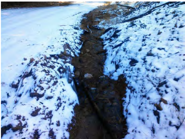
Photo 31. Non-vegetated ditch (data point 50). Orientation: west.
