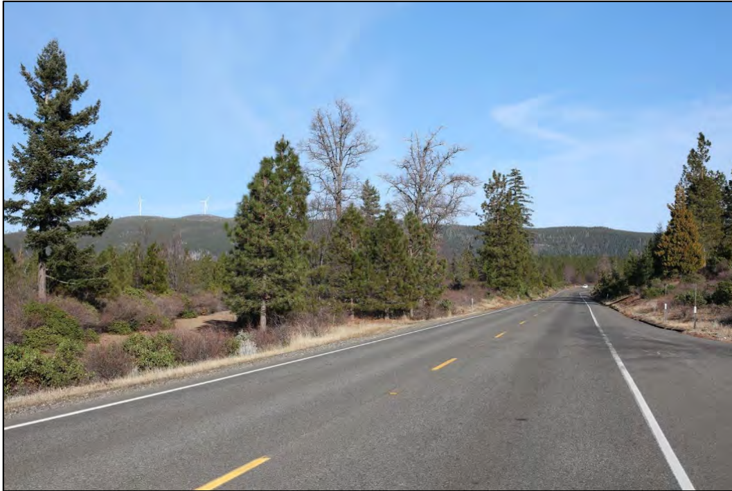
Character View 1: View along eastbound SR 299, approaching Hatchet Summit from the west. Hatchet Ridge Wind project turbines are visible to the northeast; however, most views from the highway corridor are obstructed by trees.
