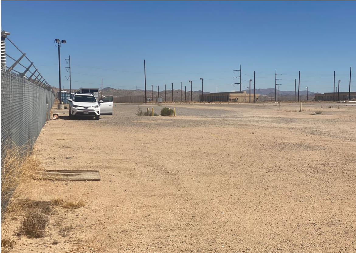
Figure 1. Photograph of HDPP Concrete Storage and Oil Containment Pad (Photograph from September 2022 looking east across Site)
