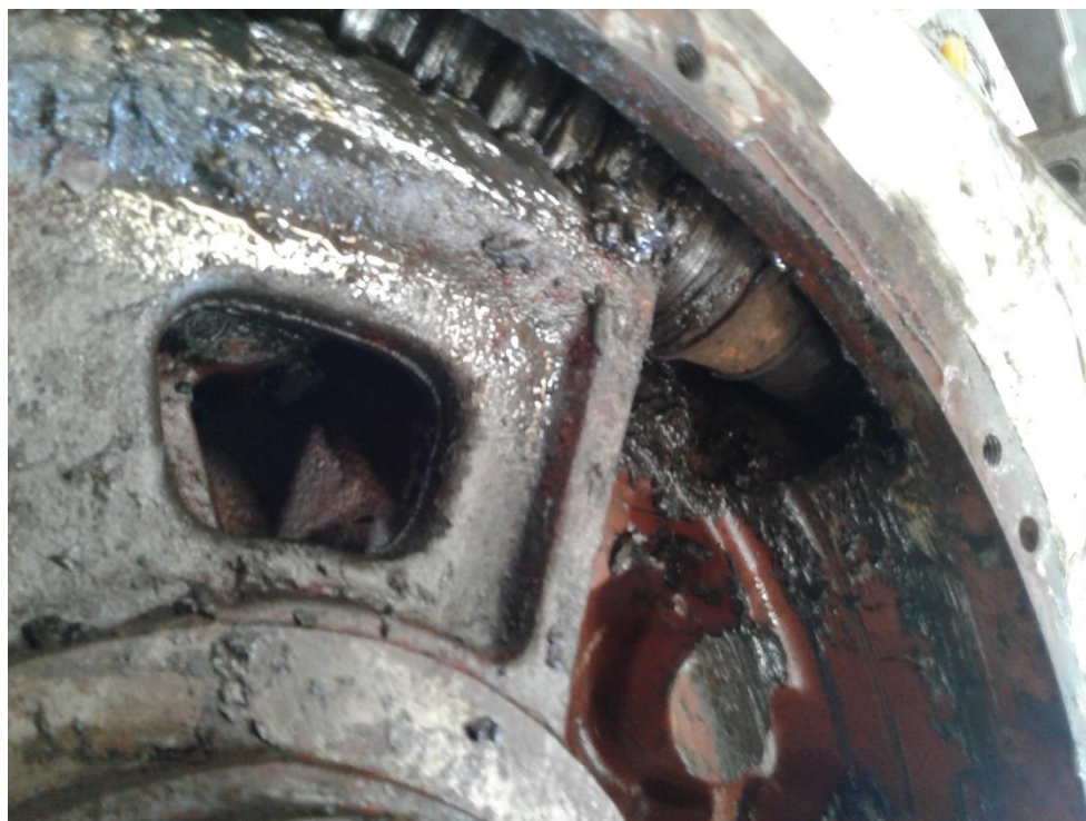
Figure 36. Additional images from the Bay Valves service center showing the disassembled gearbox.
