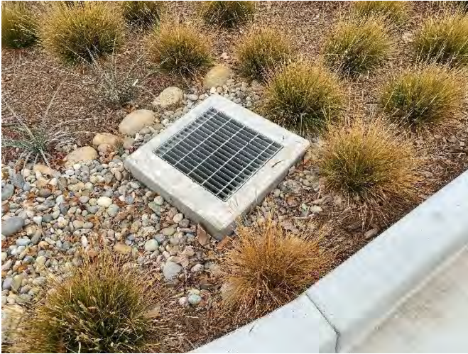
Photo 57: Catch basin inlets in Lumileds east side parking lot landscaping.
