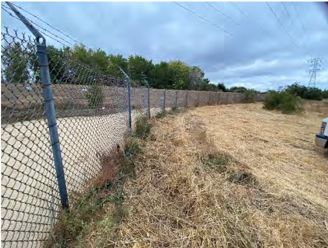
Photo 31: Looking south at south end of Property. A public sidewalk is located on top of the levee.
