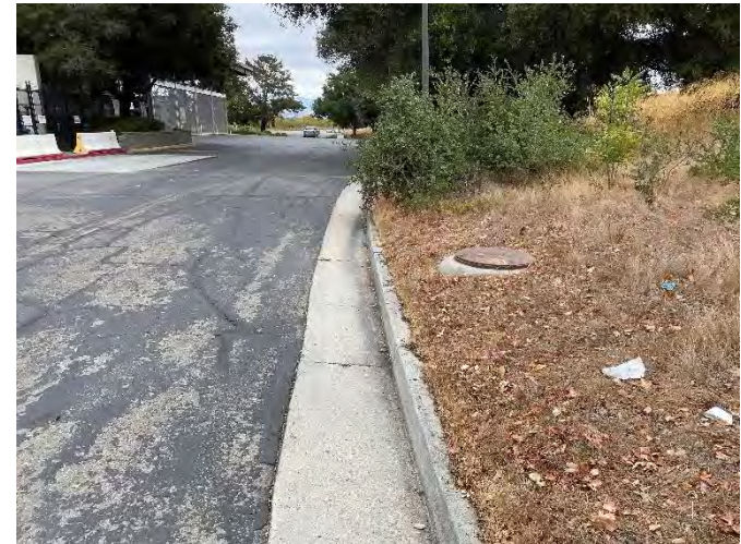
Photo 54: Looking east at sanitary sewer manhole. South side of Lumileds & north facing slope of 'hill'.
