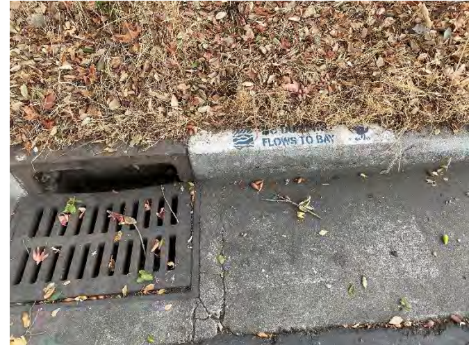
Photo 50: Closeup of catch basin inlet.
