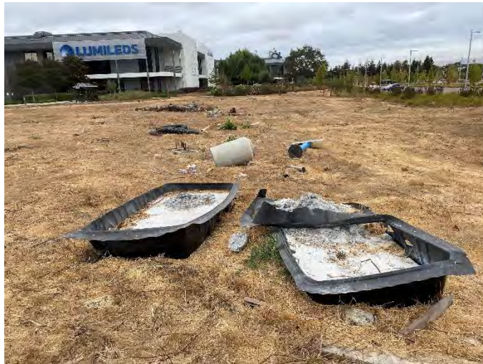
Photo 5: Concrete washout waste located on site.
