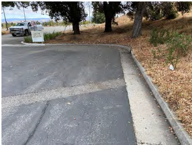
Photo 51: Looking east at storm water catch basin inlet. Property line between Lumileds and Property (south side of Lumileds).
