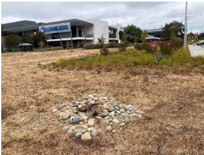
Photo 7: Looking northwest at on site catch basin inlet, maintained/non-maintained landscaping.
