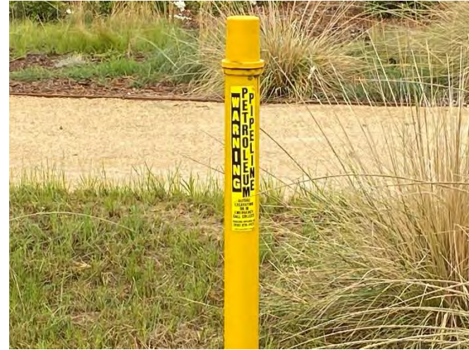
Photo 30: Close up of offsite petroleum pipeline marker. Pipeline runs northeast to southwest.
