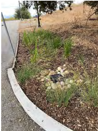
Photo 47: Looking east at storm water catch basin inlet. Property line between Lumileds and Property (south side of Lumileds).
