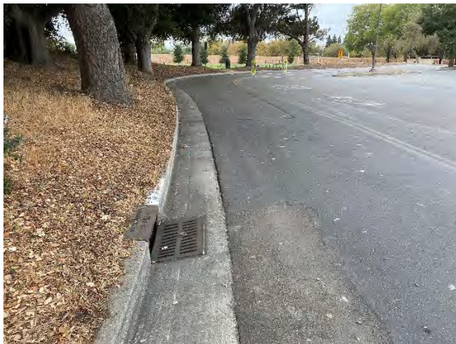
Photo 55: Looking northwest in Lumileds parking lot- stormwater catch basin inlet, north facing slope of 'hill'. Park and football field in the top center.
