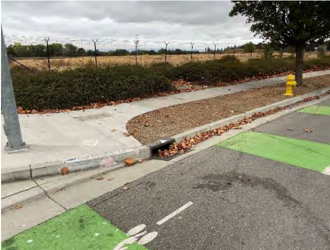
Photo 17: Looking west at stormwater inlet (off site). East corner of Property at Component Dr.
