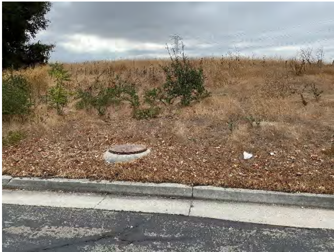
Photo 53: Looking south at sanitary sewer manhole on north facing slope of 'hill'.
