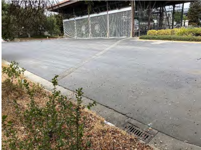
Photo 49: Looking northeast from storm water catch basin inlet at Lumileds ASTs.
