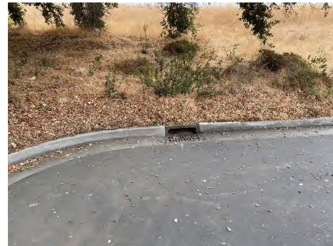
Photo 48: Offsite- Looking south at storm water catch basin inlet. South side of Lumileds, north facing slope from 'hill'.
