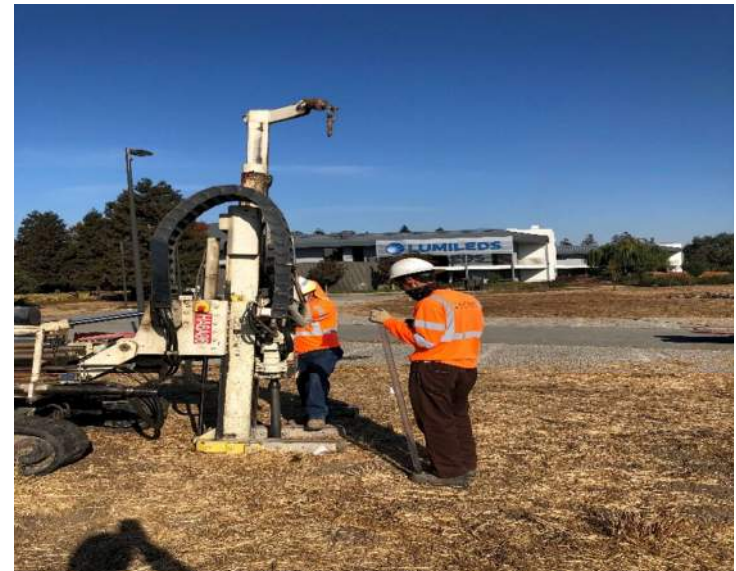
Photo 10: (SP-2) Direct push drilling to 20 feet bgs.
