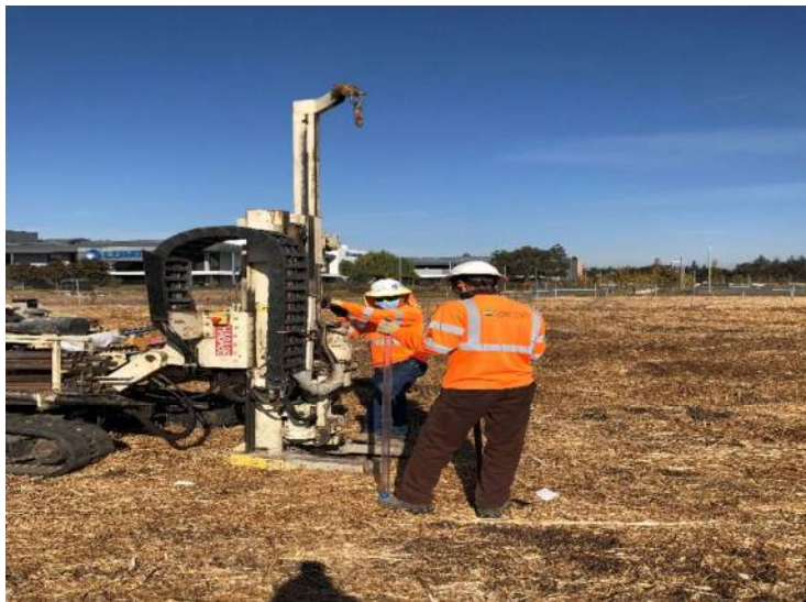
Photo 11: (SP-3) Direct push drilling to 20 feet bgs.
