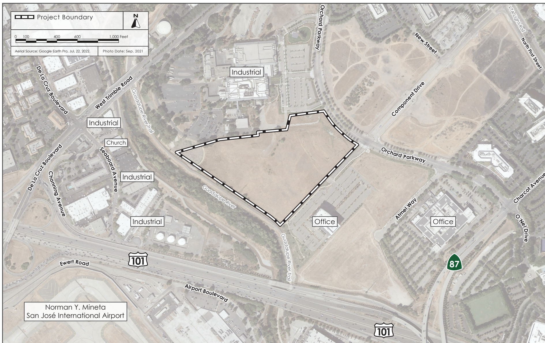
AERIAL PHOTOGRAPH AND SURROUNDING LAND USES
