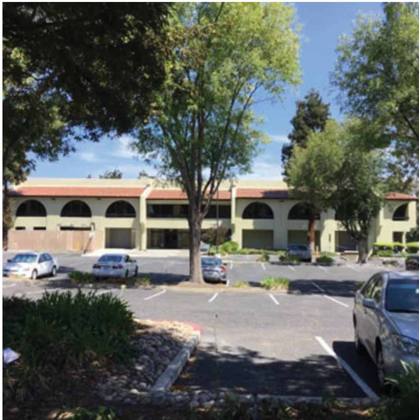
Photo 2: The south elevation of 2805 Bowers Avenue, view North
