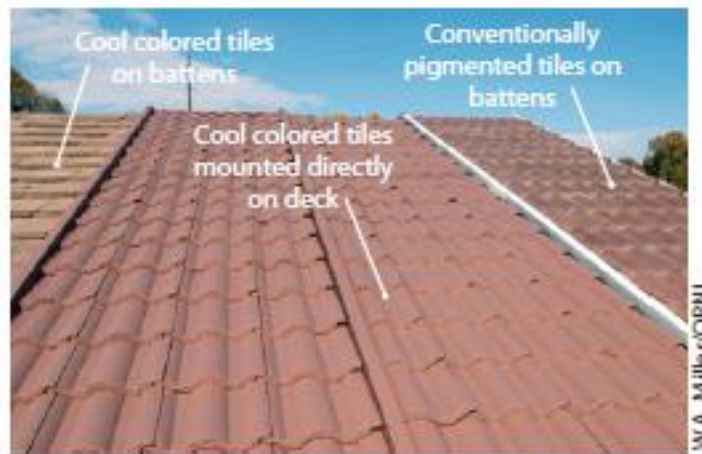
Figure 2. Conventional and Cool Colored Tiles (EPA 2011)
