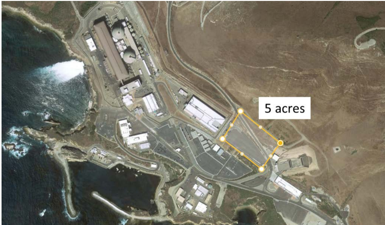
Figure 2-16: Land areas projected onto satellite images of the area near Diablo Canyon. We note that the projected areas are not actual proposed plant sites, but are strictly meant to convey the scale of different project footprints
