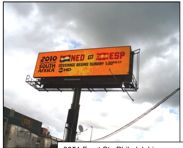
3051 Front St., Philadelphia Off-premise LED sign
