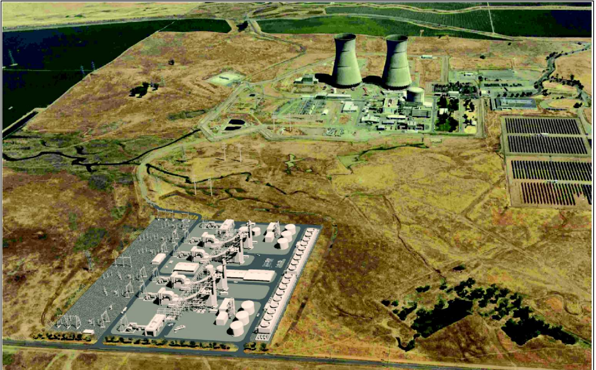
FIGURE 1.1-5R APPEARANCE OF THE SITE AFTER CONSTRUCTION, LOOKING NORTH COSUMNES POWER PLANT APPLICATION FOR CERTIFICATION
