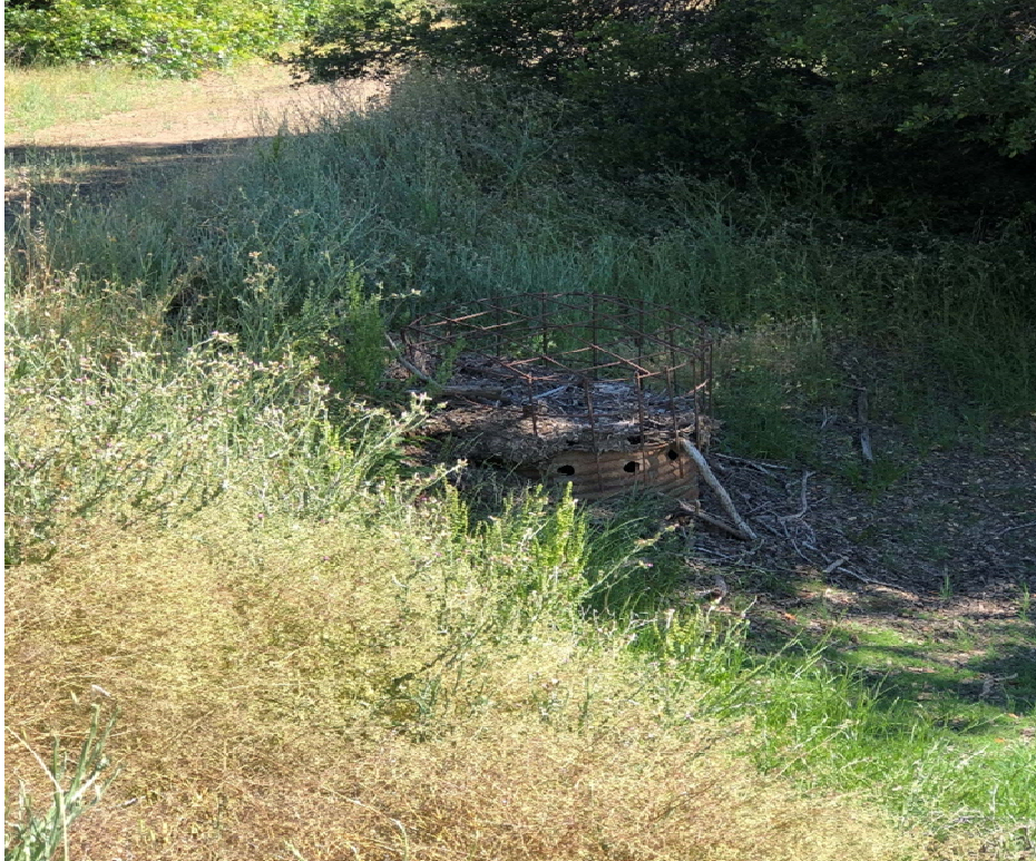
U17 Pond – Overflow Functional, but Pond is Dry.
