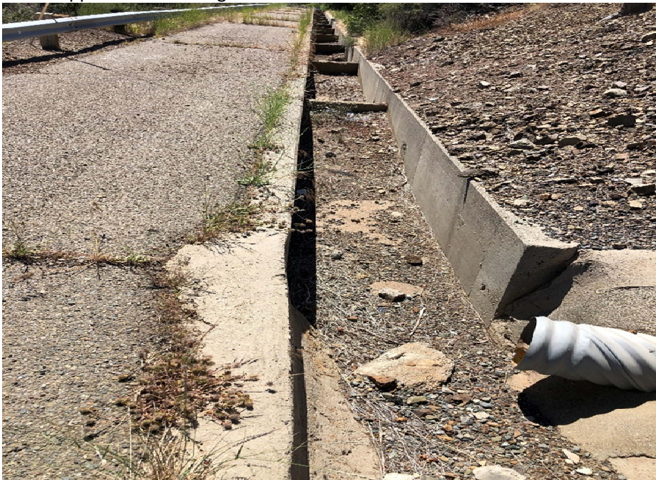
Sonoma Dams have gravel in top few sections needing to be cleaned to prepare for next rainy season. Gravel appears to be falling in from road above.
