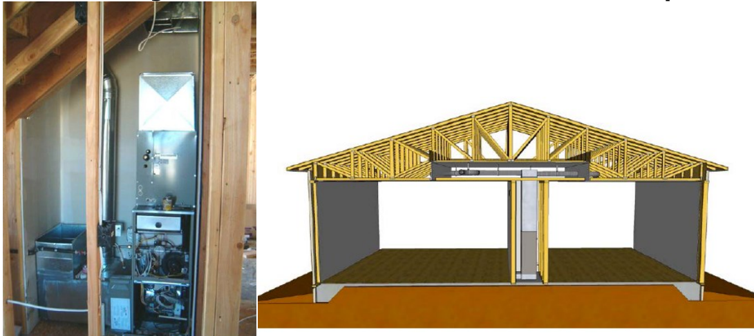
Figure 4-14: Mechanical Closet Placement Example
