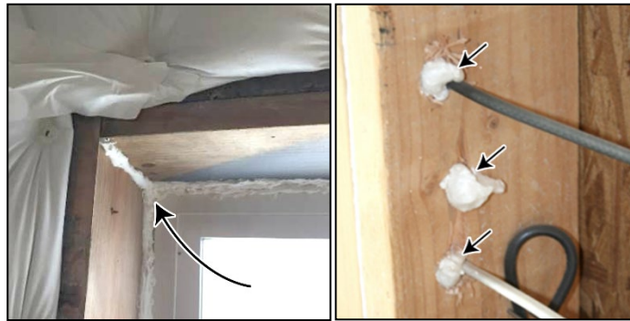
Figure 3-10: Air Sealing
