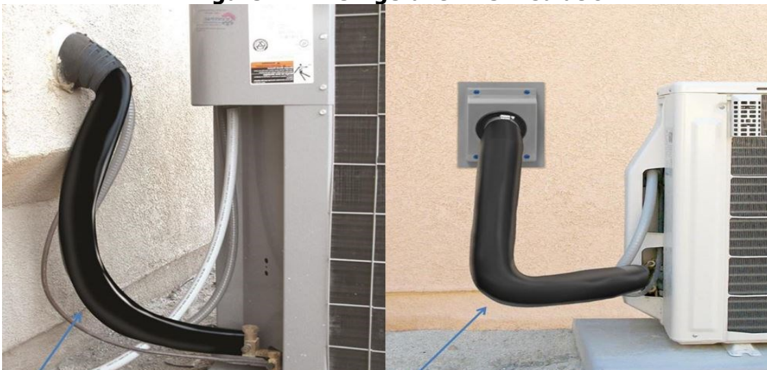
Figure 4-1: Refrigerant Line Insulation
