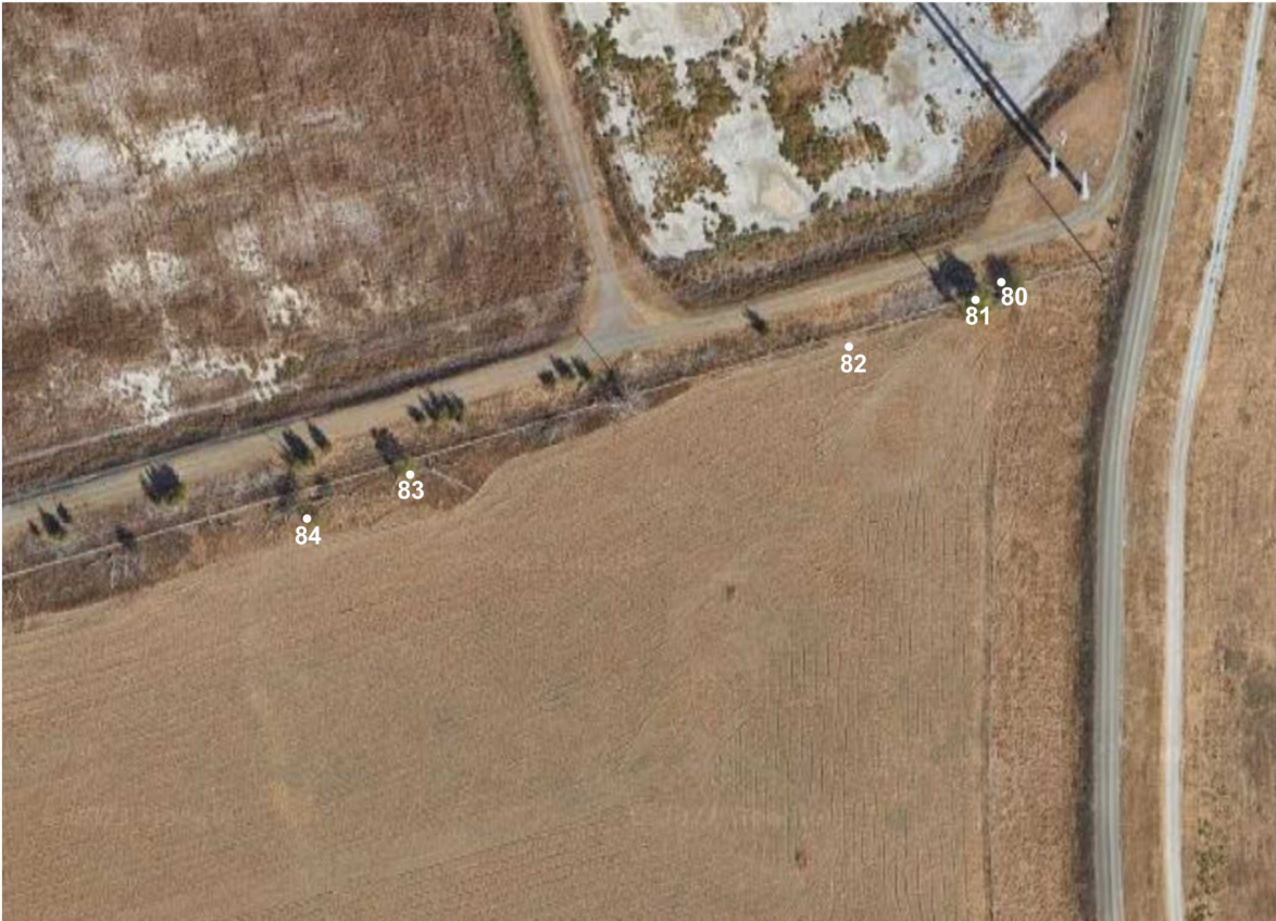
TREES #80-84: Northernmost property line are recommended for removal.
