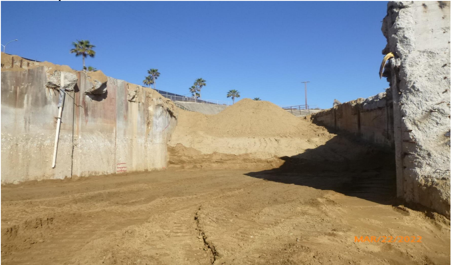
Photo #10 Imported Soil backfill at north end of Channels
