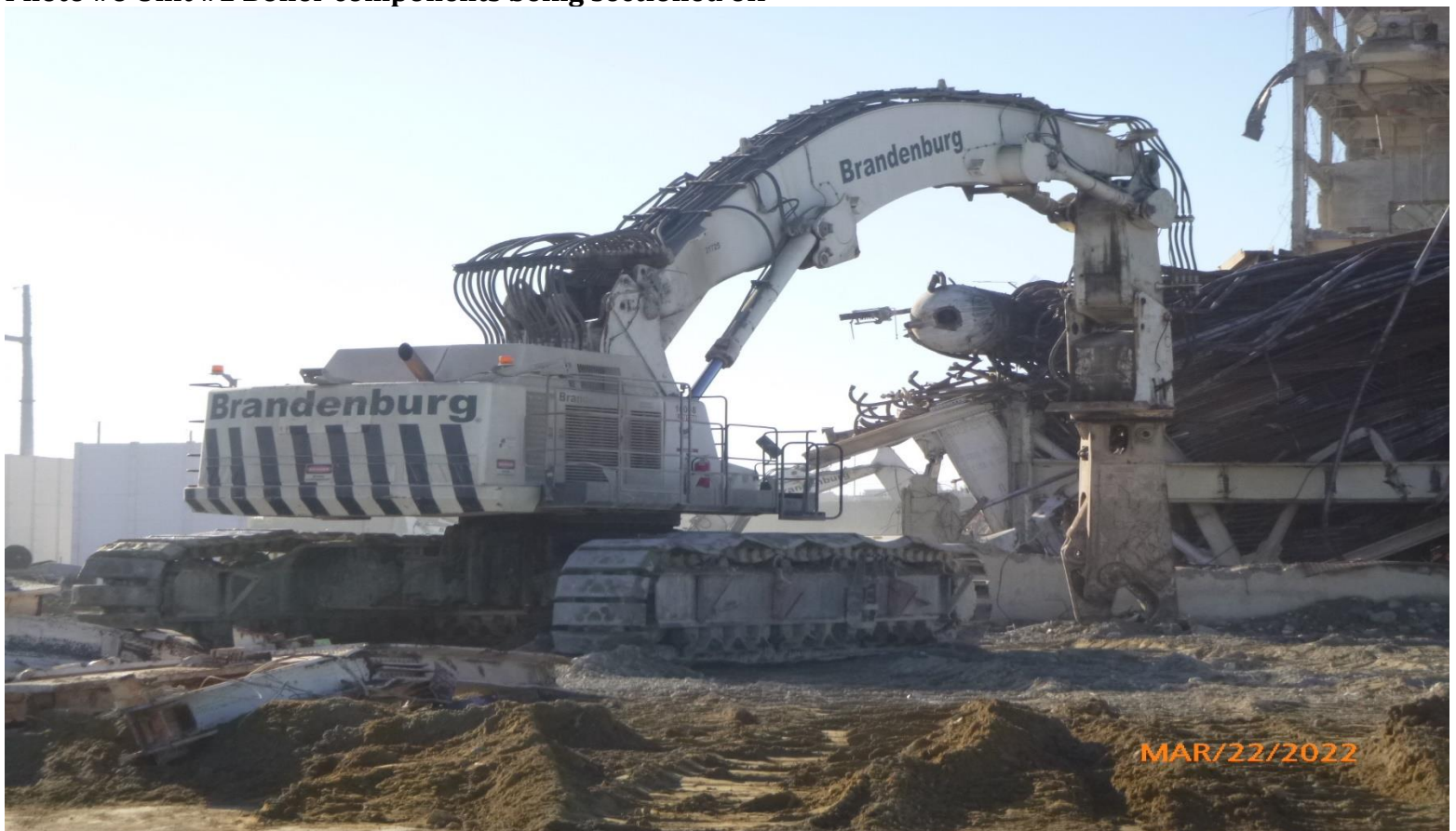
Photo #6 Unit #1 Boiler components being sectioned off
