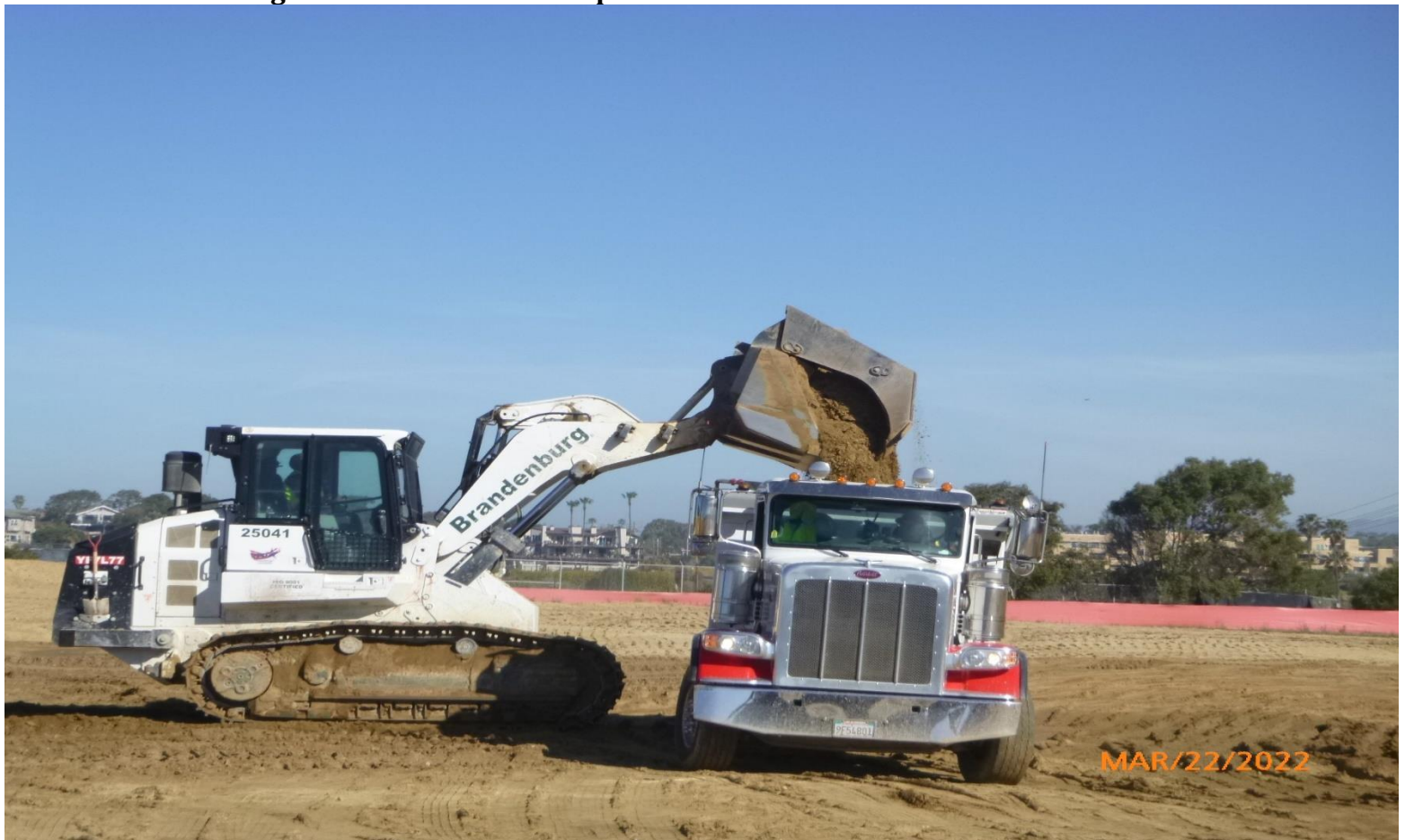
Photo #12 Retrieving Soil backfill from Stockpile Site.
