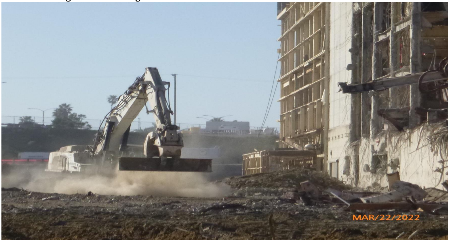
Photo #14 Using steel beams to grade and clean demo areas
