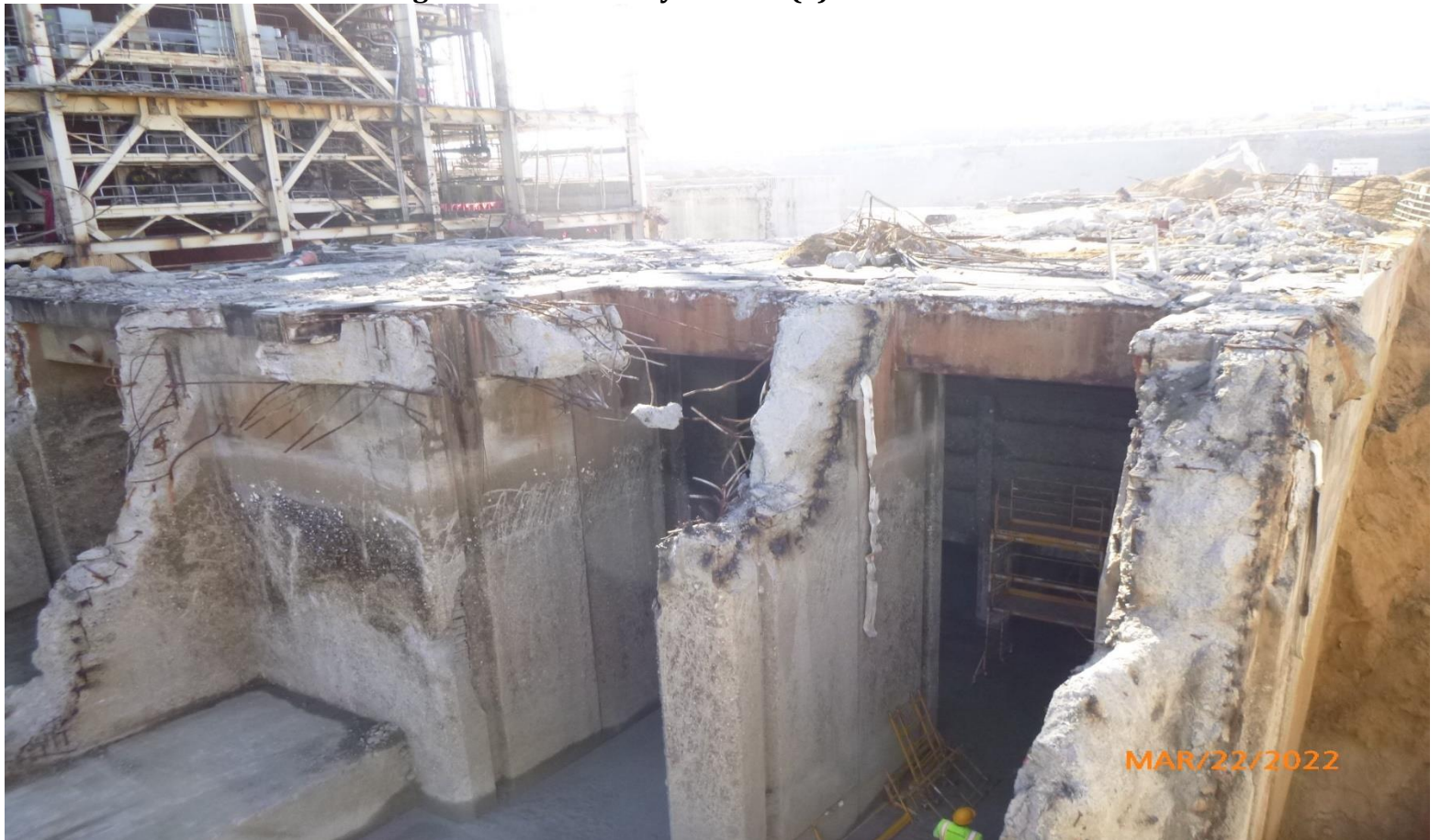
Photo #8 Water Channels being cleaned for slurry backfill (a)
