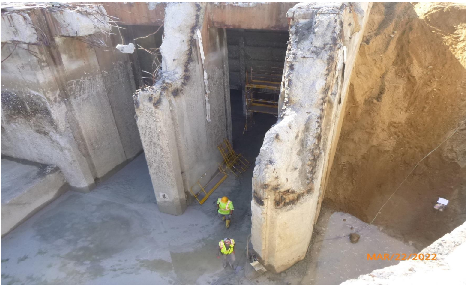
Photo #10 Imported Soil backfill at north end of Channels
