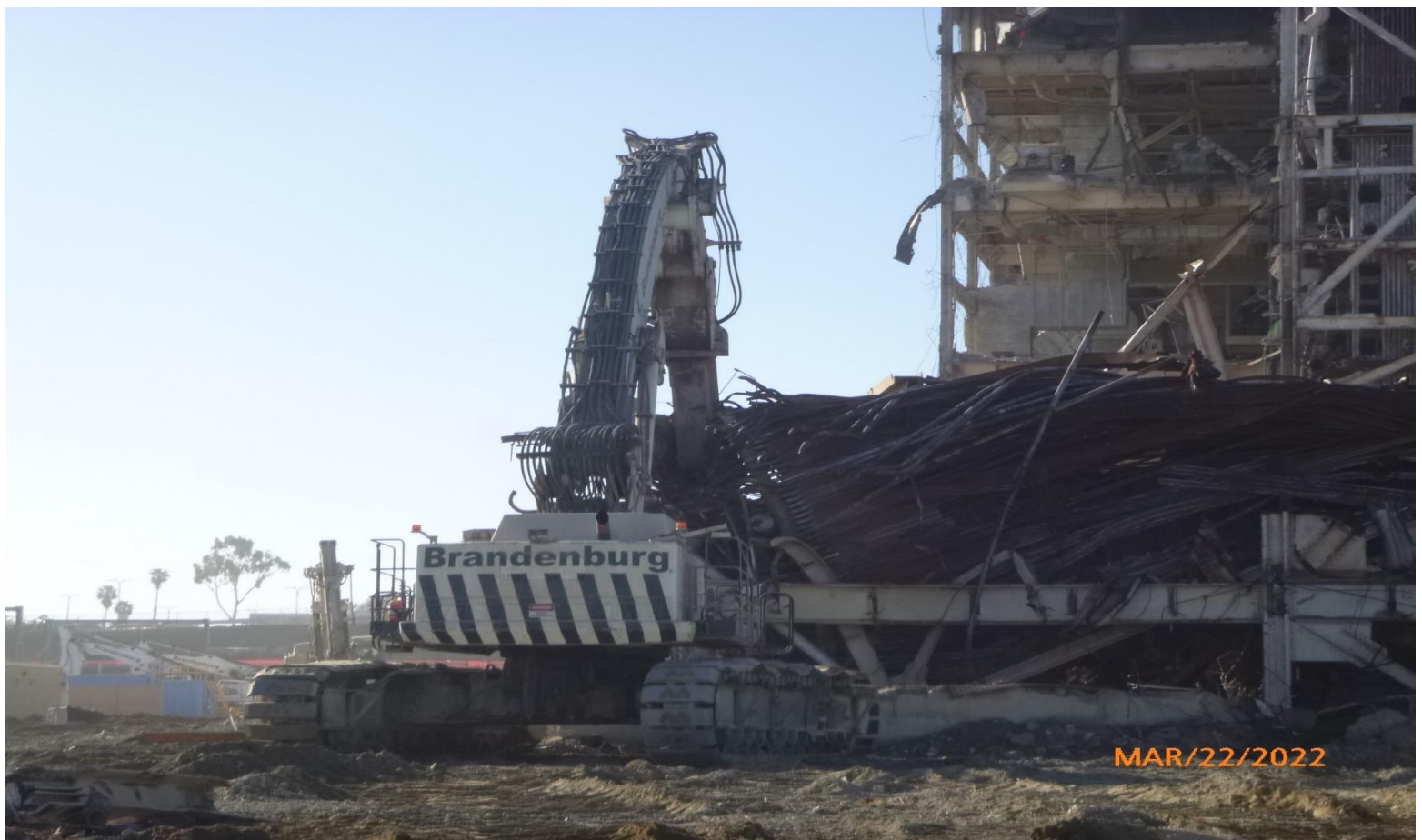
Photo #6 Unit #1 Boiler components being sectioned off
