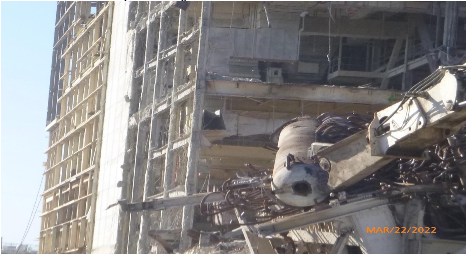
Photo #2 Unit#1 Boiler Components being removed
