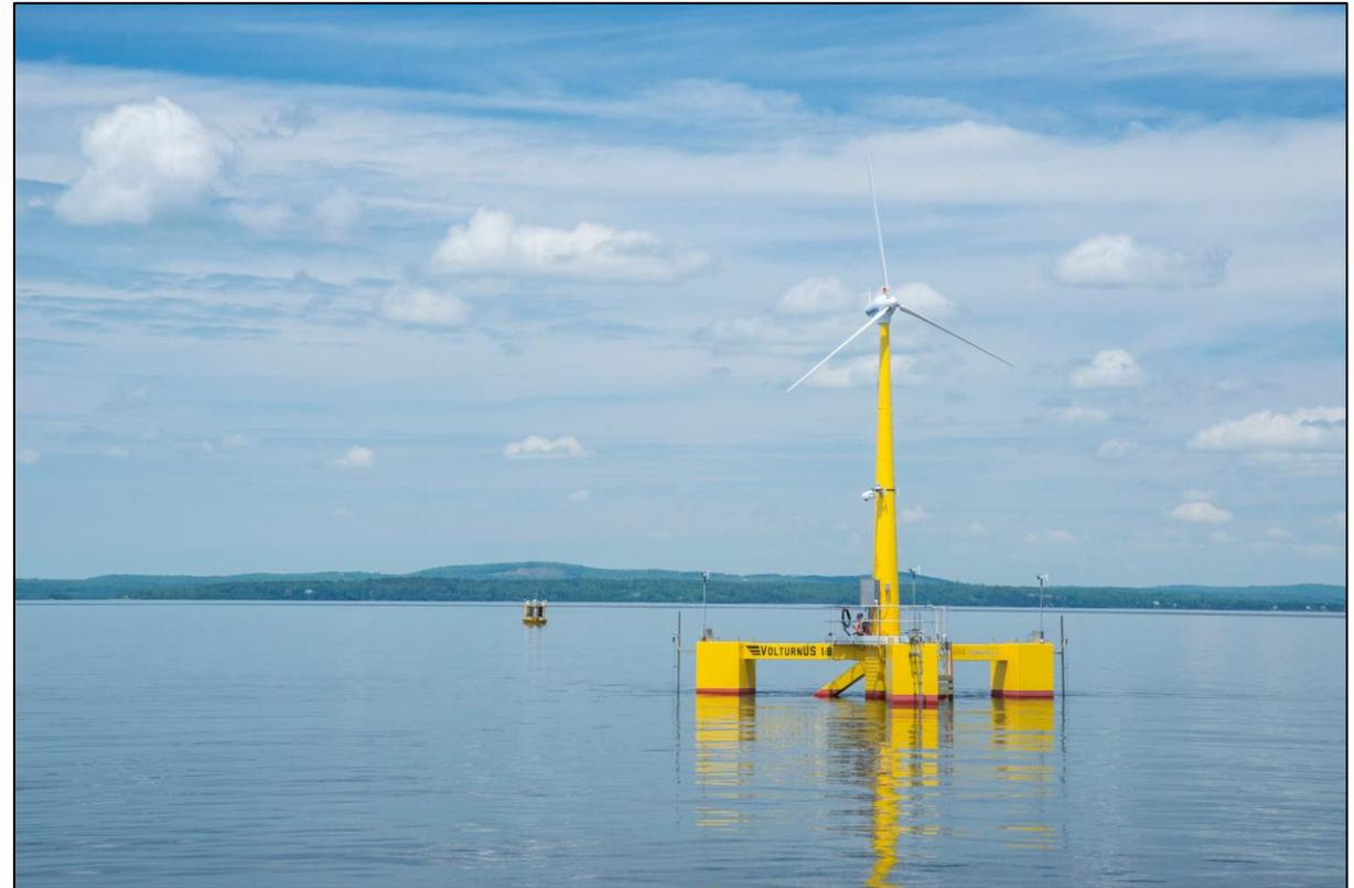
VoltturnUS, 1:8 scale of a 6 MW wind turbine near Maine. VoltturnUS was built at U Maine. It is the first grid connected offshore wind turbine in the US. (<https://composites.umaine.edu/research/voltturnus/>)
