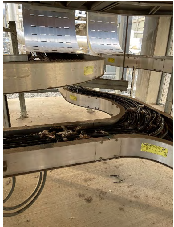
Cable tray under the Power Distribution Center
