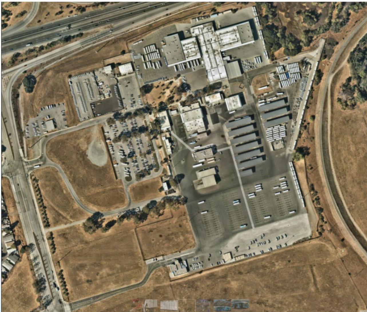
Aerial View of Santa Clara Valley Transportation Authority Site
