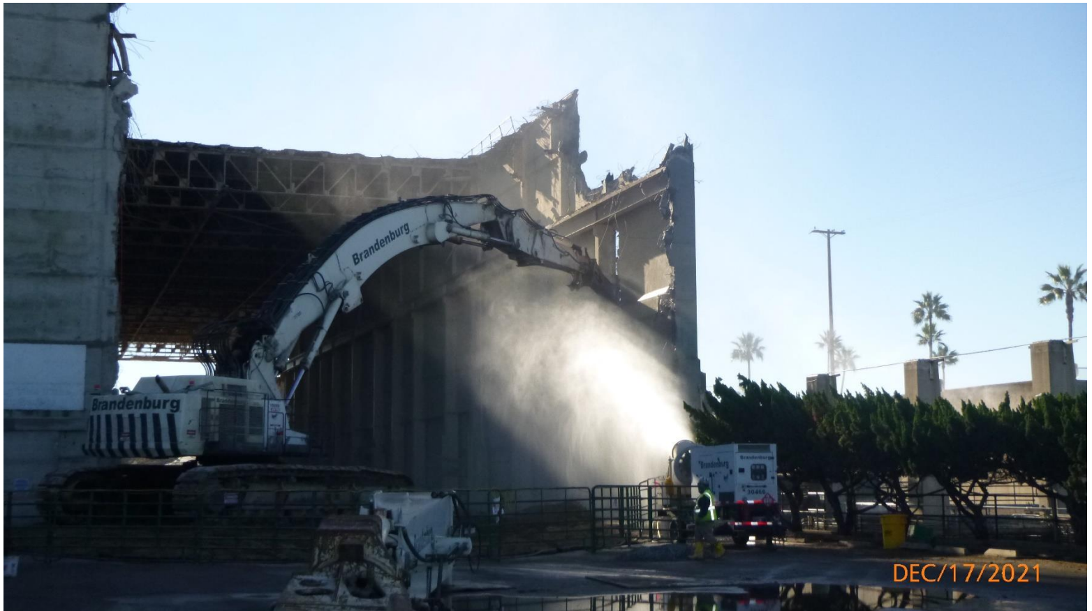
Photo #12: Demo of Concrete Panels note water misters for dust control
