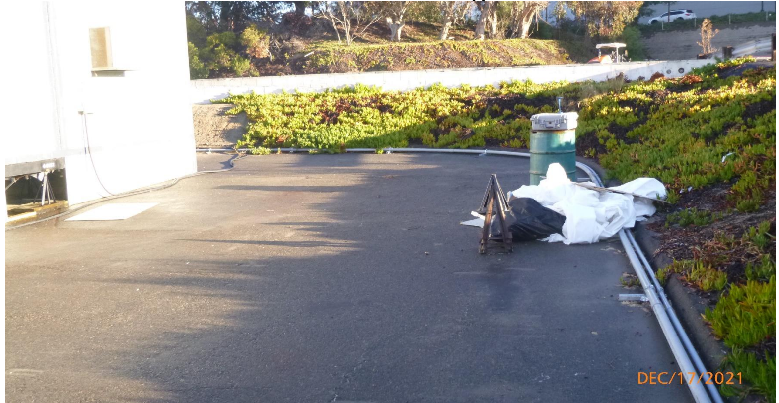
Photo #1: Service Conduits from MDB to Trailers secured and supported PVC
