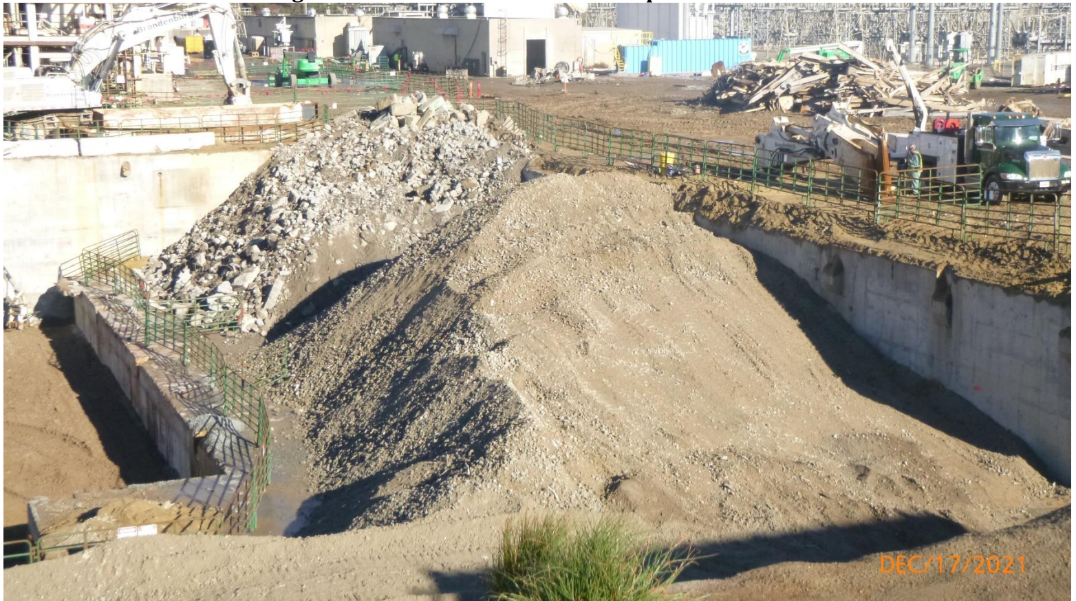
Photo #13: Backfill material generated from crushed concrete operations.
