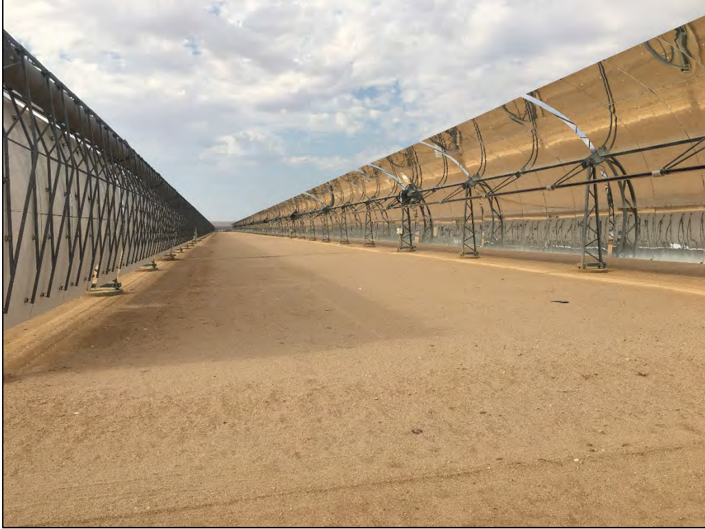
Photo 1: Panels of Site 5
