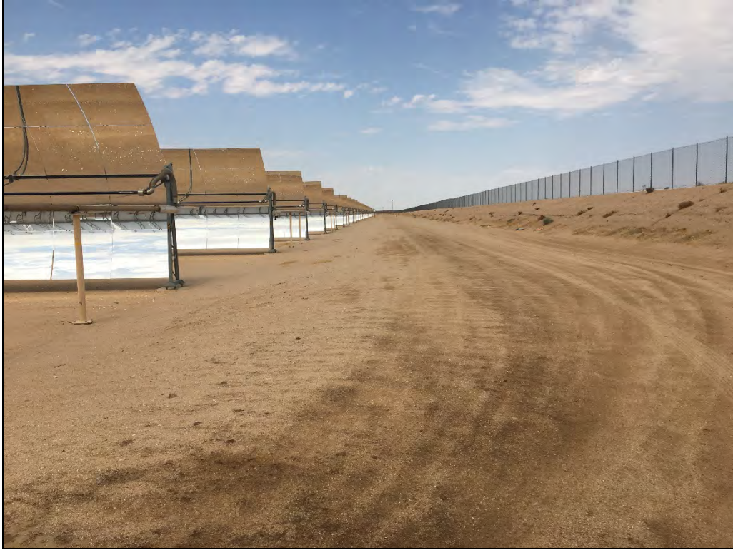
Photo 7: Northeast corner of Site 6 looking west.
