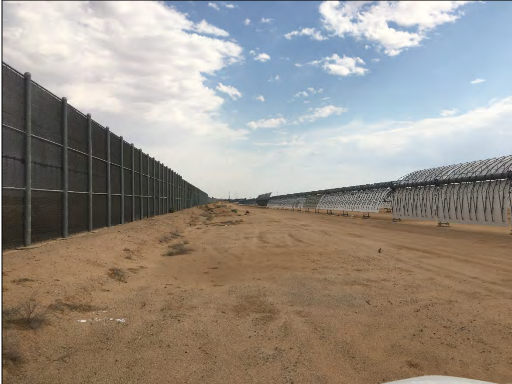
Photo 2: Southwest corner of Site 4 looking north.
