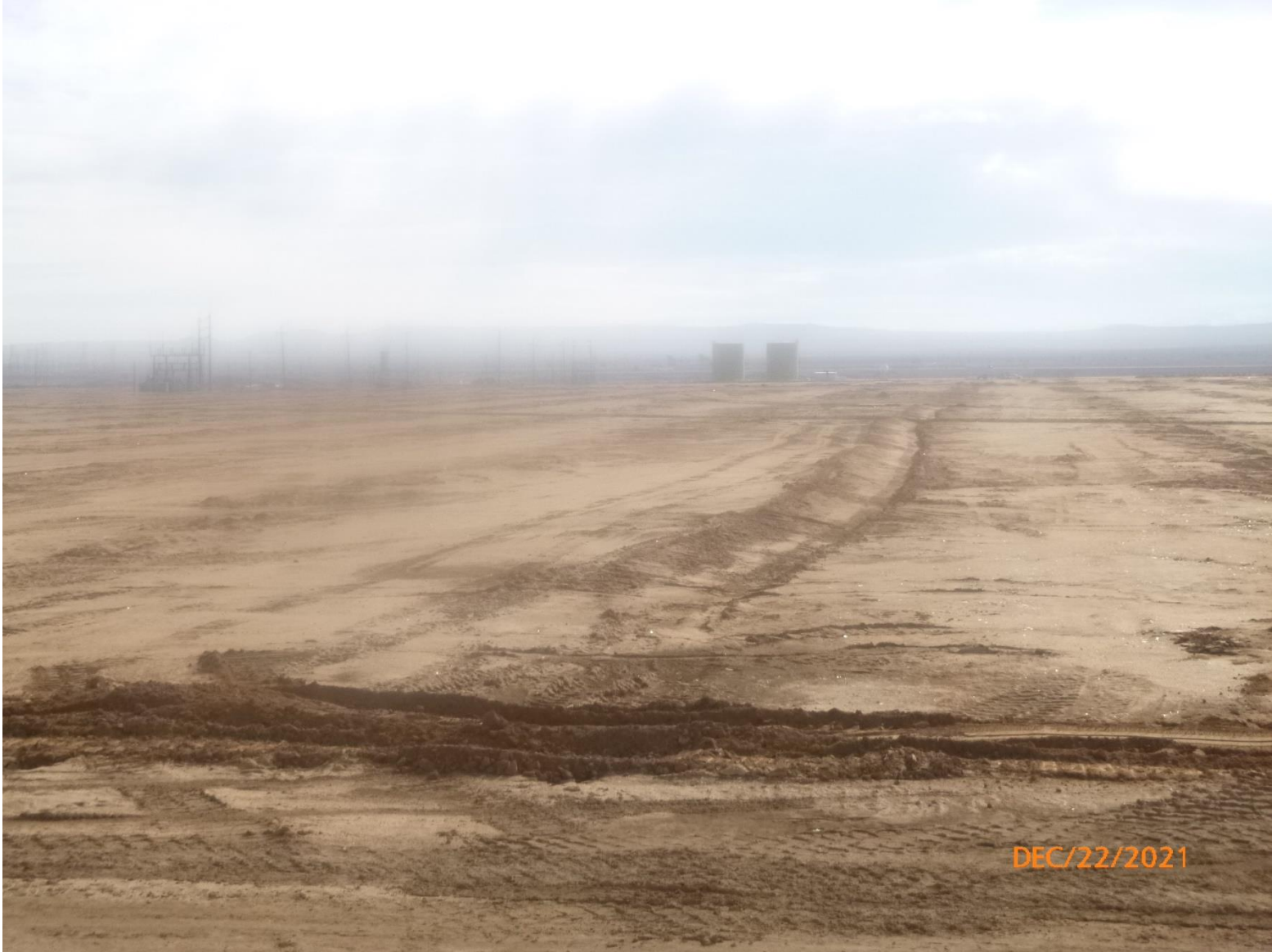
#8 SEGS V viewed from East to West. V power block in distance
