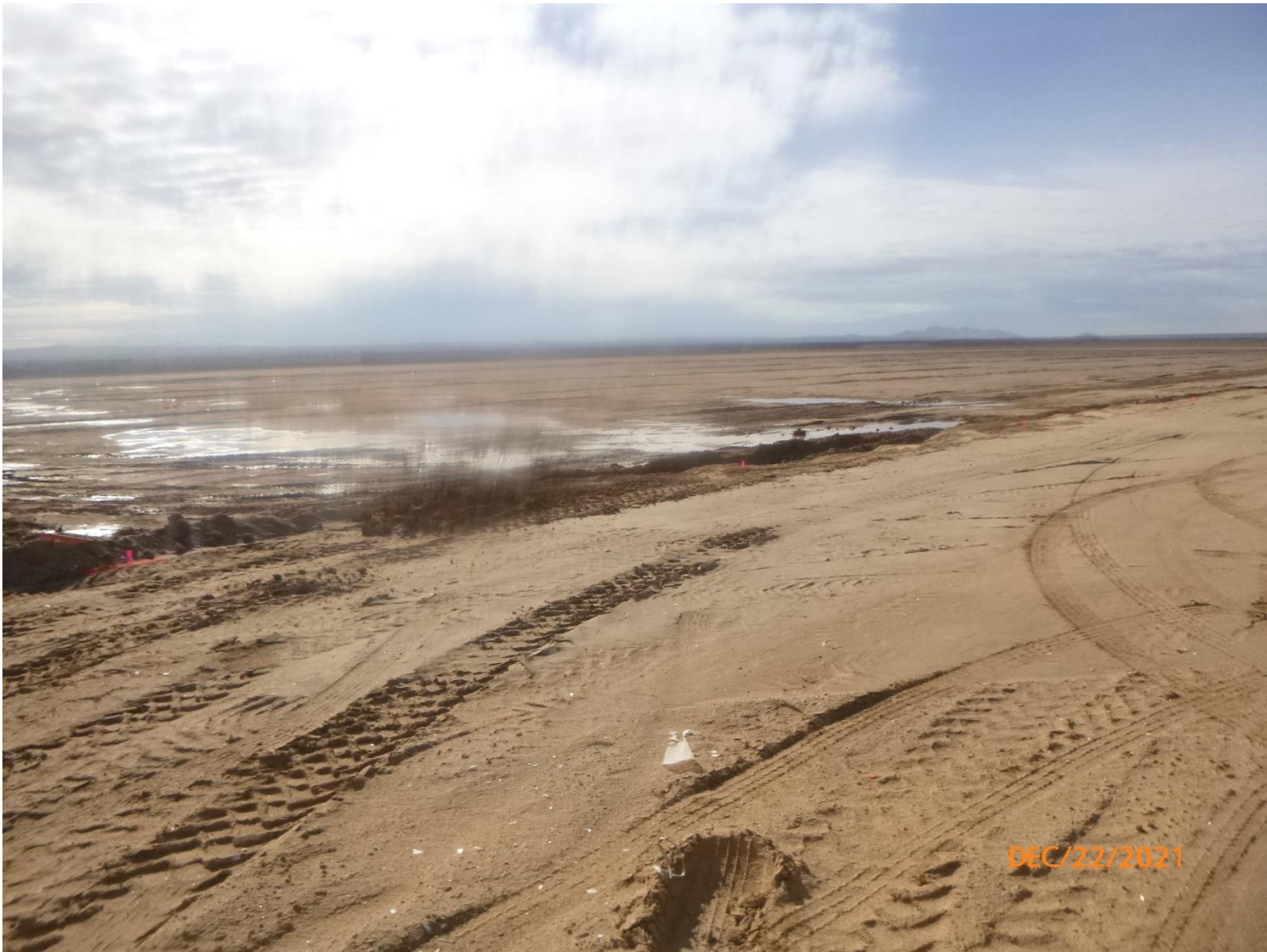
#2 SEGS III View from east to west
