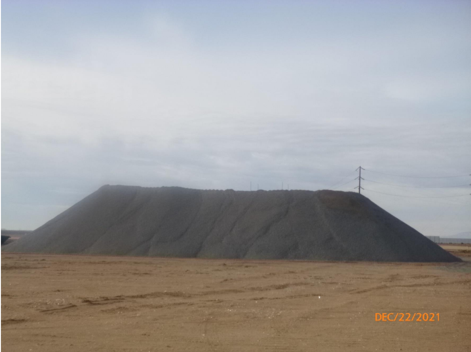
#3 SEGS IV Gravel stockpile for future construction
