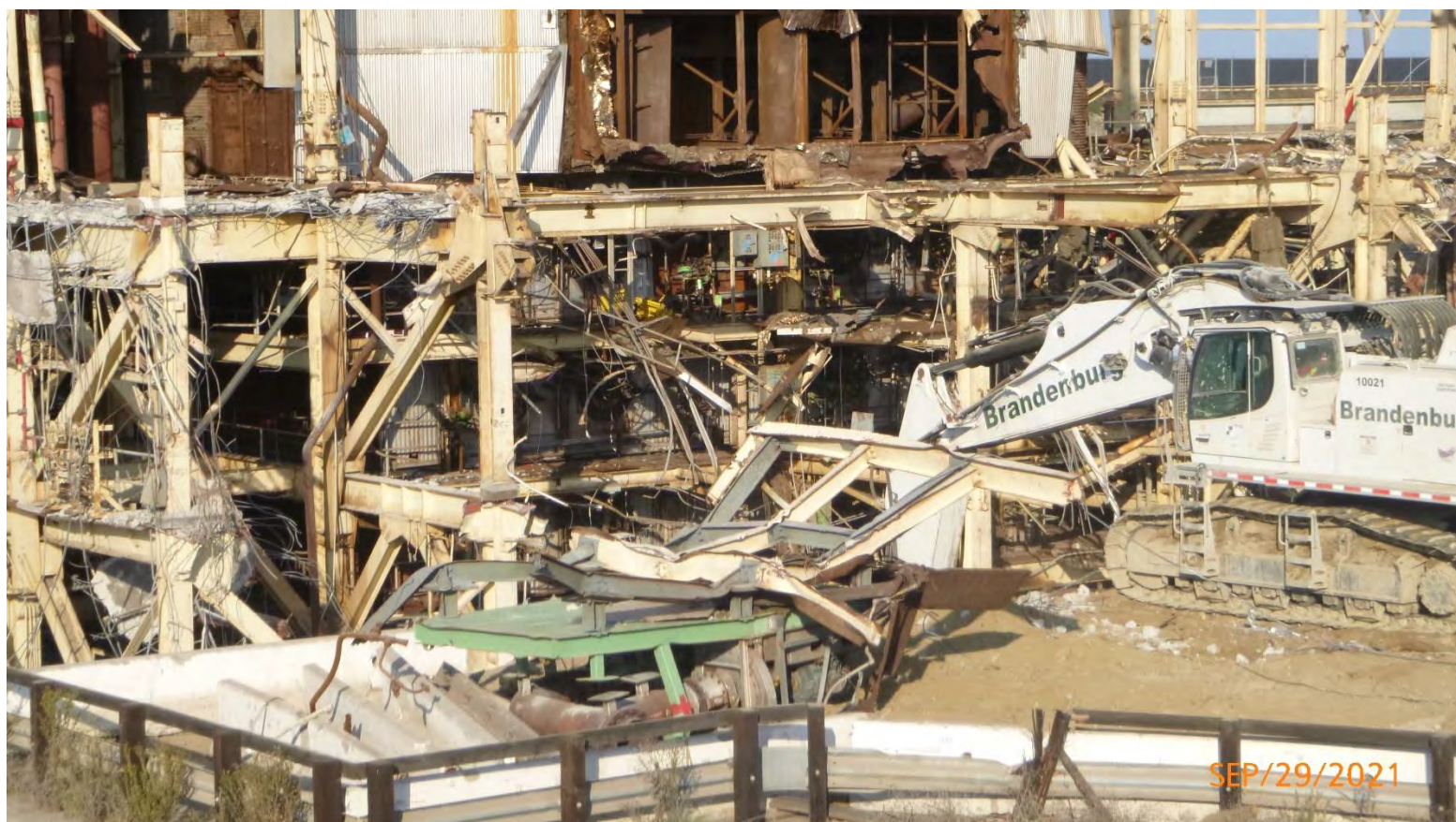
Photo #8: Unit #5 Structural demo ongoing east face. (b)
