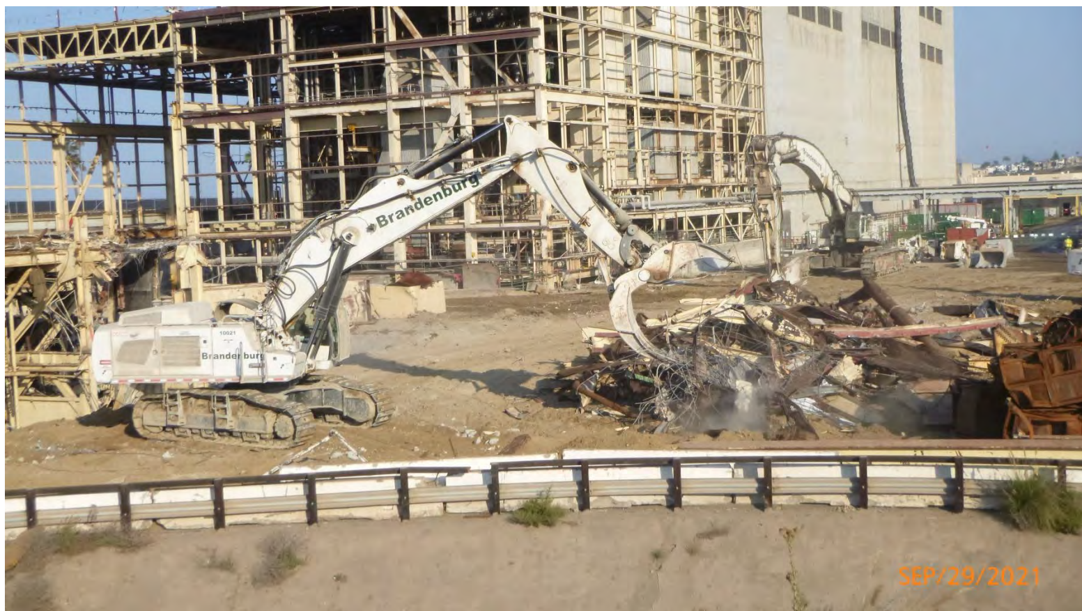
Photo #6: Separating misc. steel for recycle. (b)
