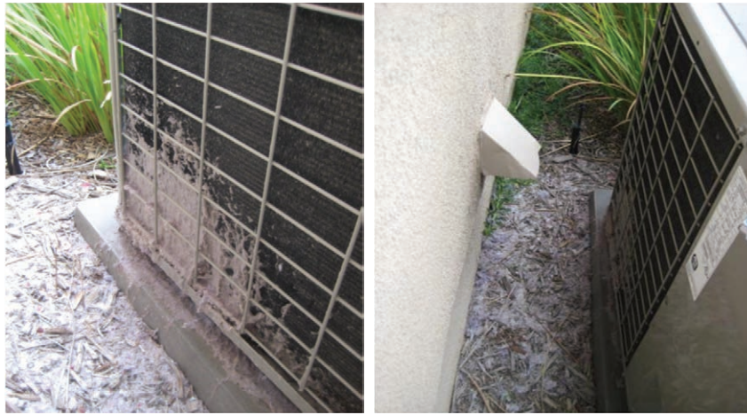
Figure 11-38: Noncompliant Condensing Unit Clearance from Dryer Vents
