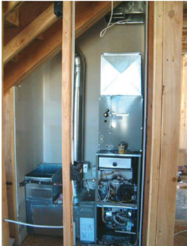
Figure 4-14: Mechanical Closet Placement Example
