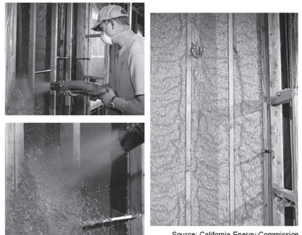
Figure 3-15: Cellulose-Insulated Wall
