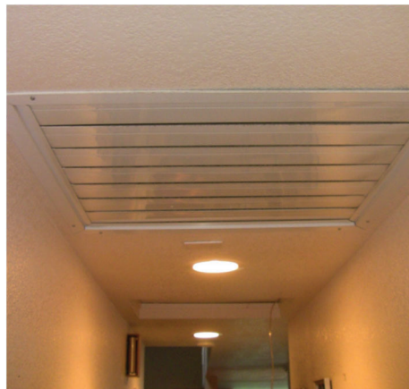
Figure 4-38: Whole-House Fan With Barometric Damper
