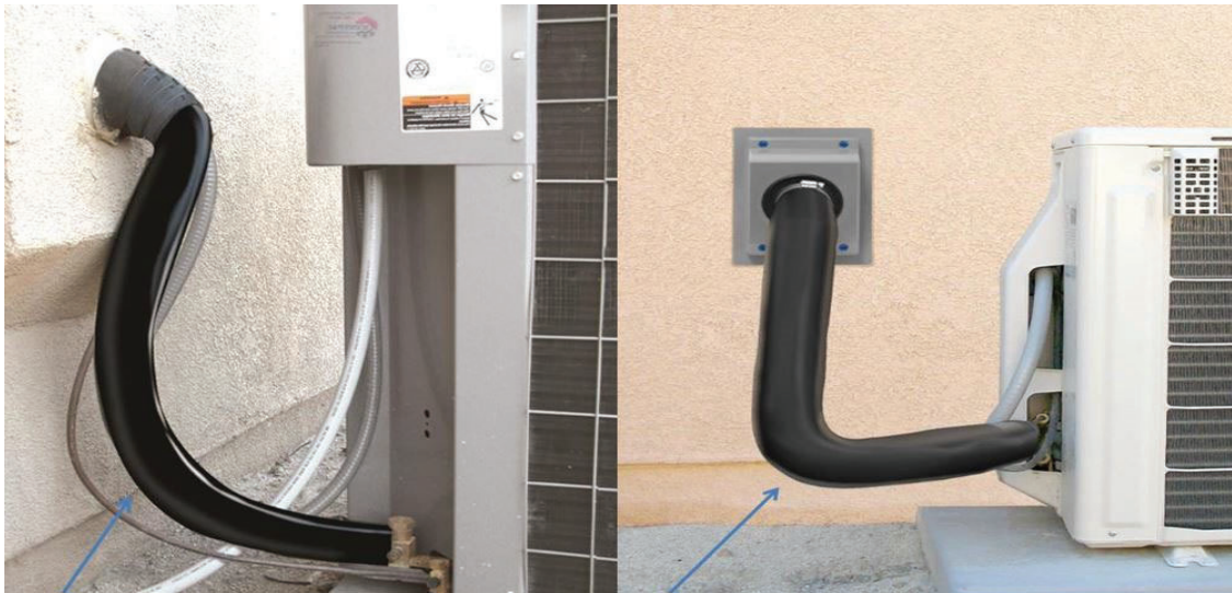
Figure 4-1: Refrigerant Line Insulation
