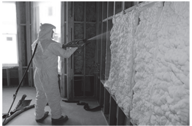
Figure 3-17: Open-Cell SPF Installed in Wall Cavity
