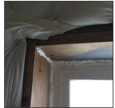
Figure 3-10: Air Sealing
