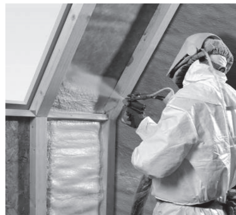
Figure 3-18: Closed-Cell SPF Installation in a Wall Cavity
