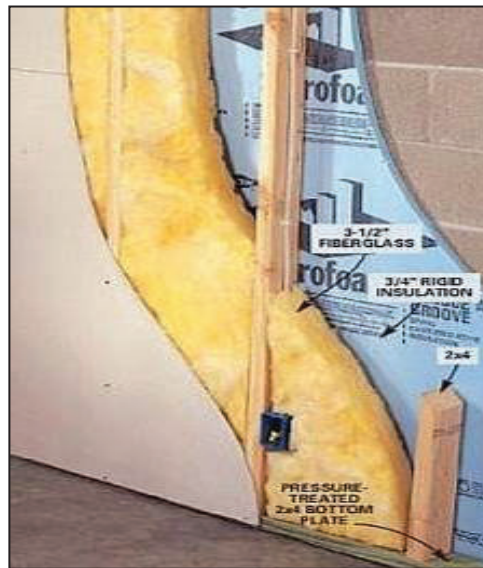
Figure 3-29: Masonry Wall With Furring Details
