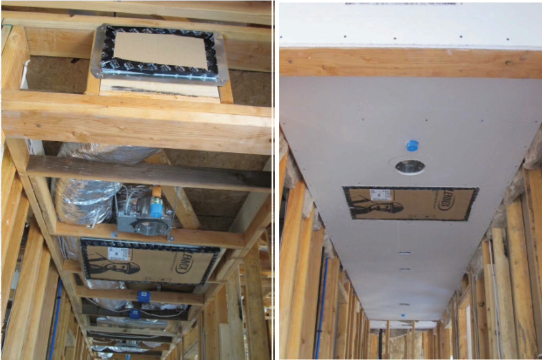
Figure 4-11: Ducts Routed Through a Dropped Ceiling
