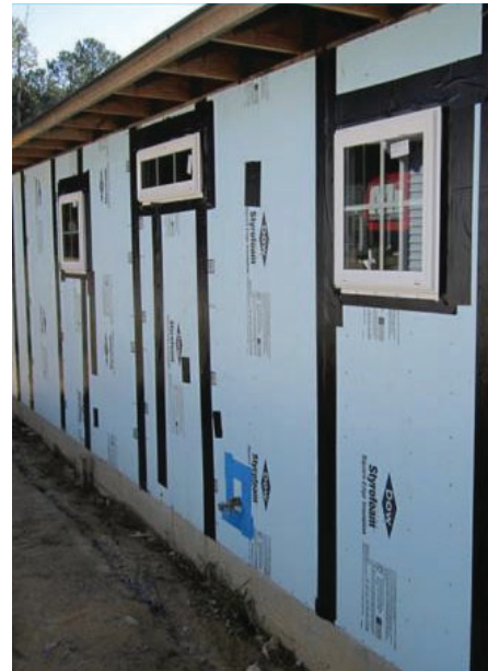
Figure 3-19: Properly Installed Rigid Insulation With Sealant Tape
