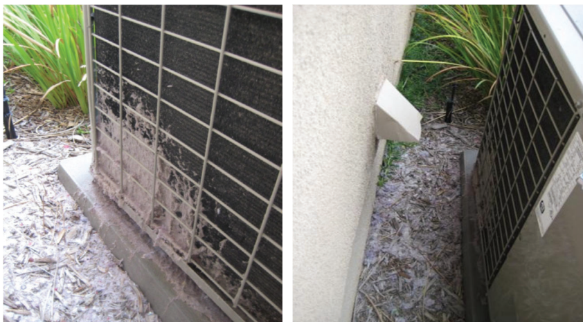
Figure 4-2: Noncompliant Condensing Unit Clearance from Dryer Vents
