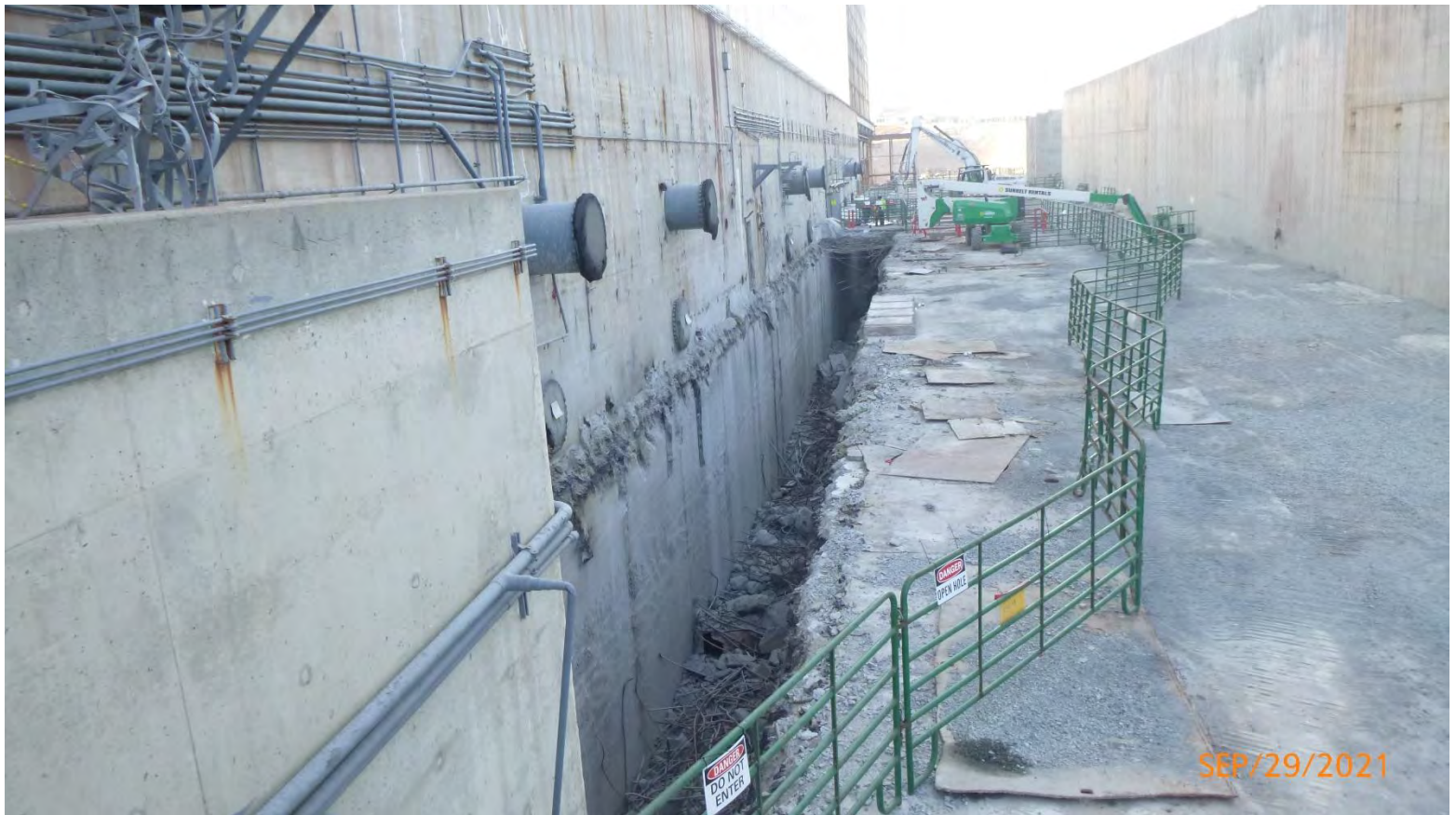
Photo #12: Exposed channel opened to backfill
