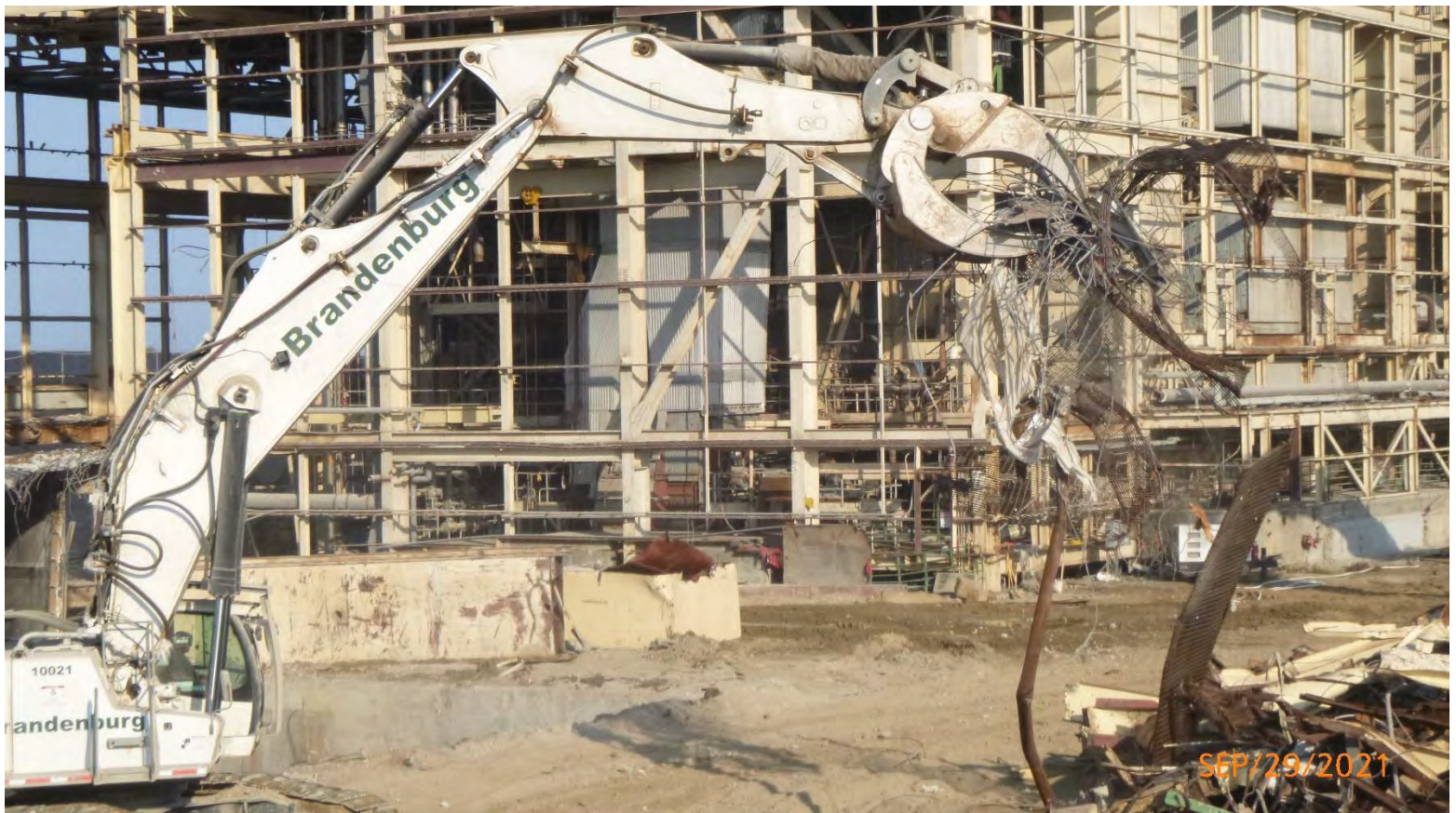
Photo #5: Separating misc. steel for recycle. (a)
