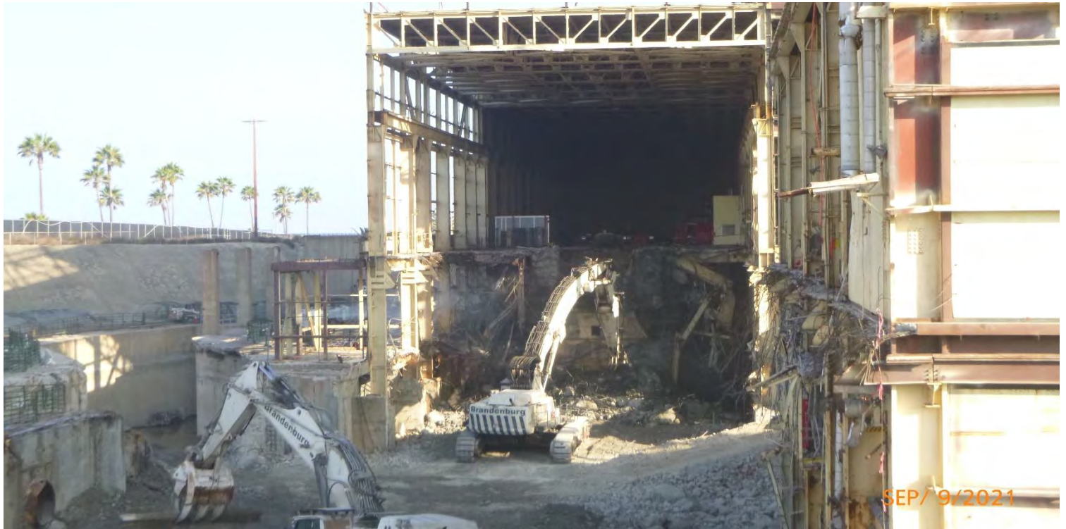
Photo #4: Demo of Foundation at Unit #4 turbine foundation
