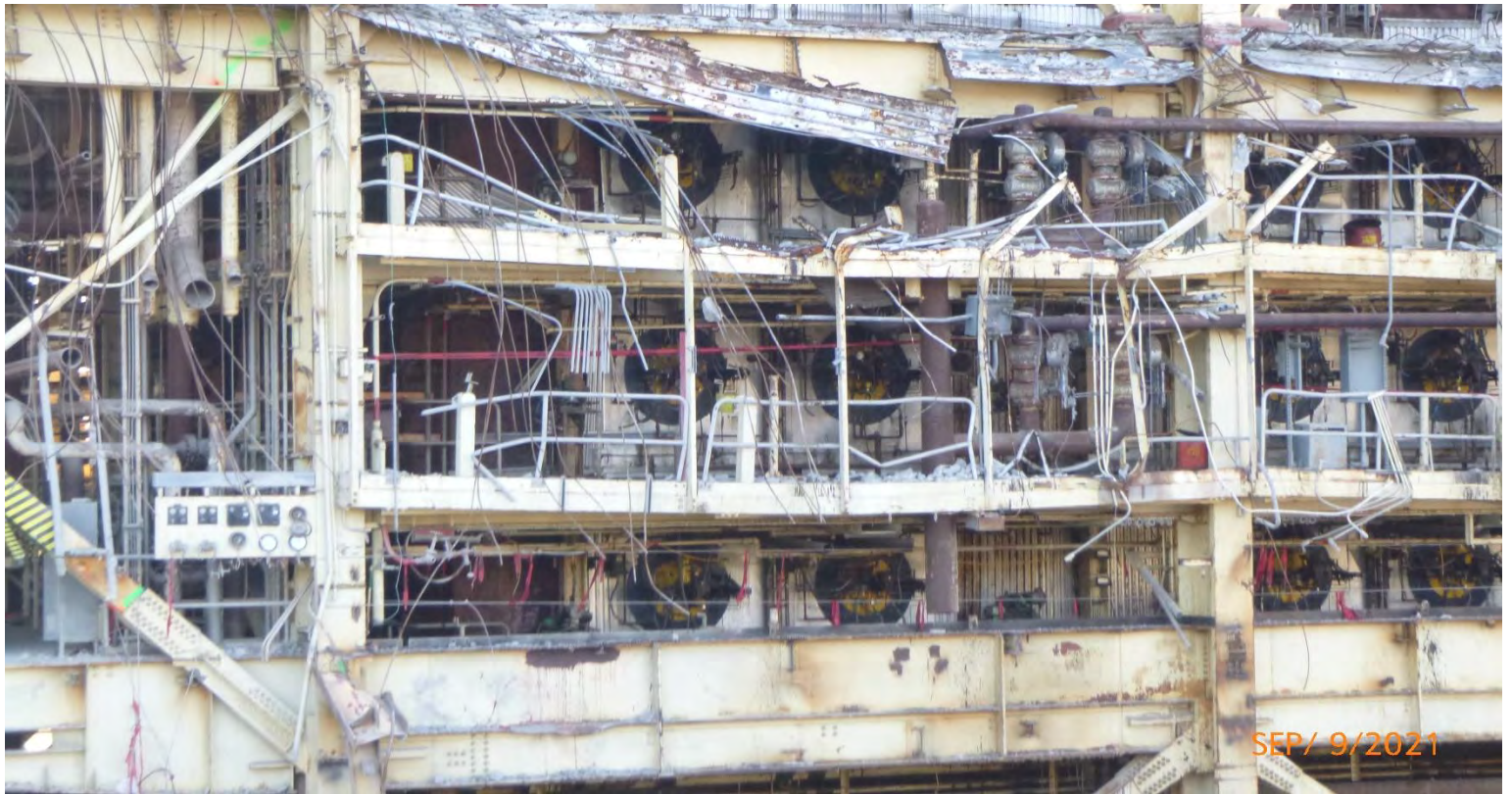
Photo #18: Interior floor levels exposed after removal of Unit#5
