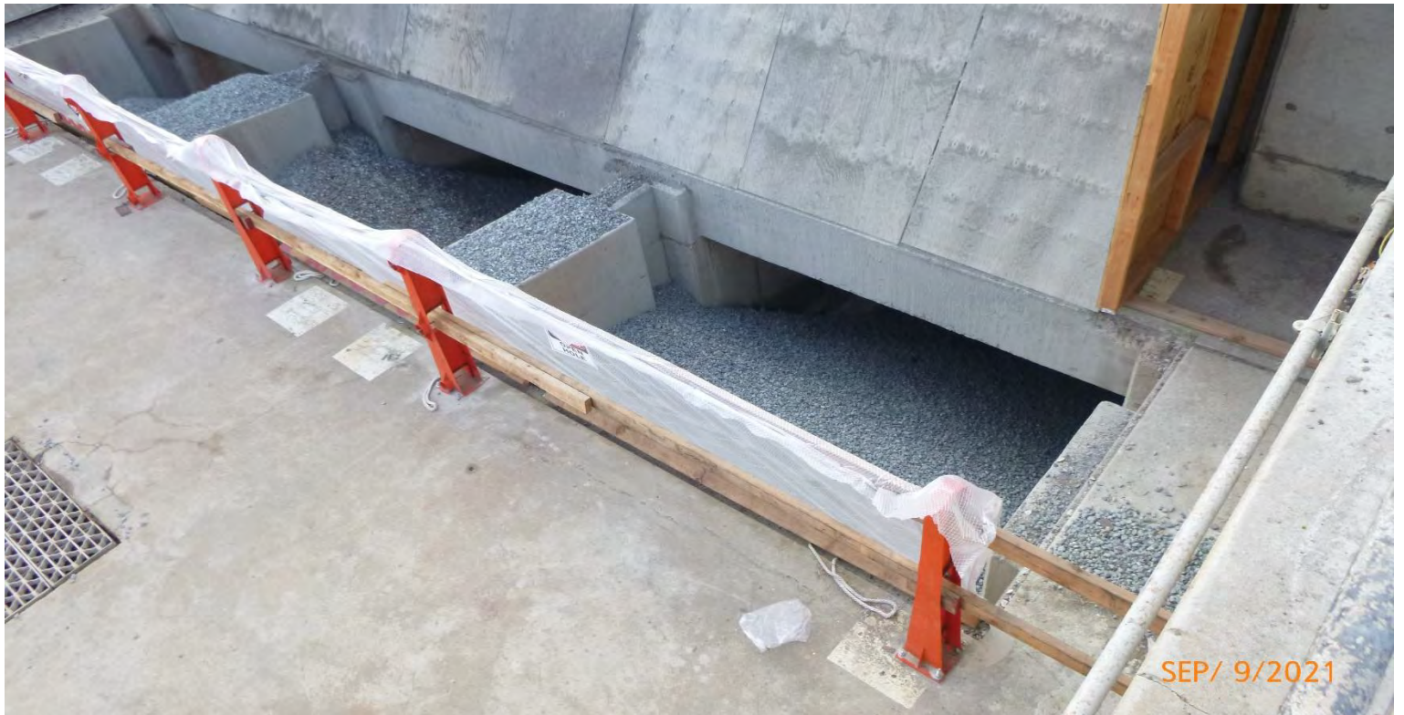
Photo #16: Water Channels ongoing backfill operations
