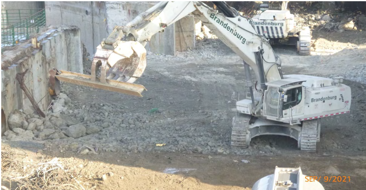
Photo #7: Demo and structural steel used as straight edge to level grade
