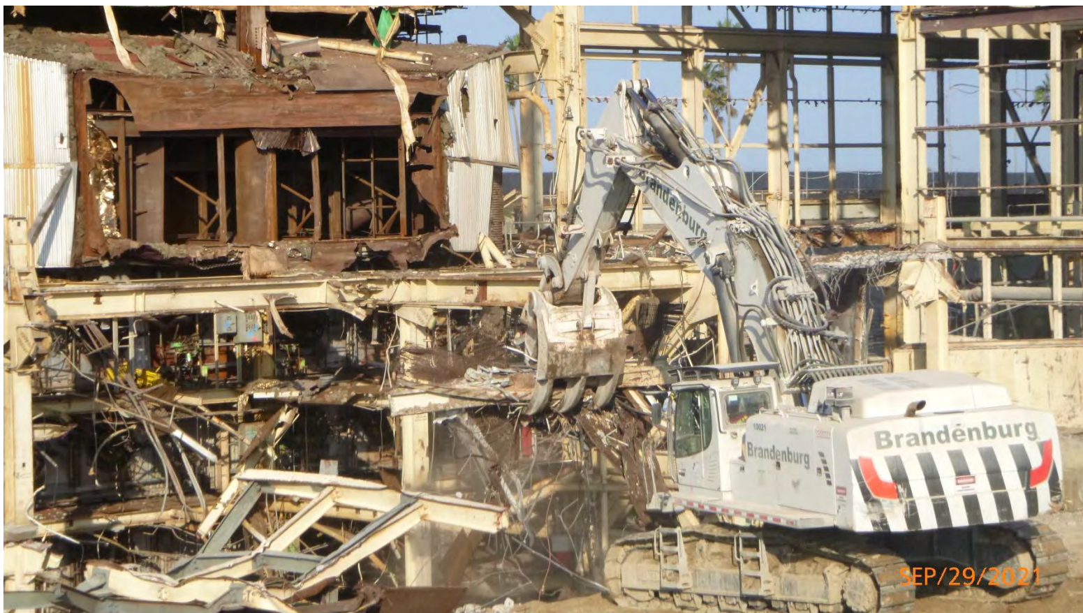
Photo #9: Unit #4 Turbine bay Fdn removed
