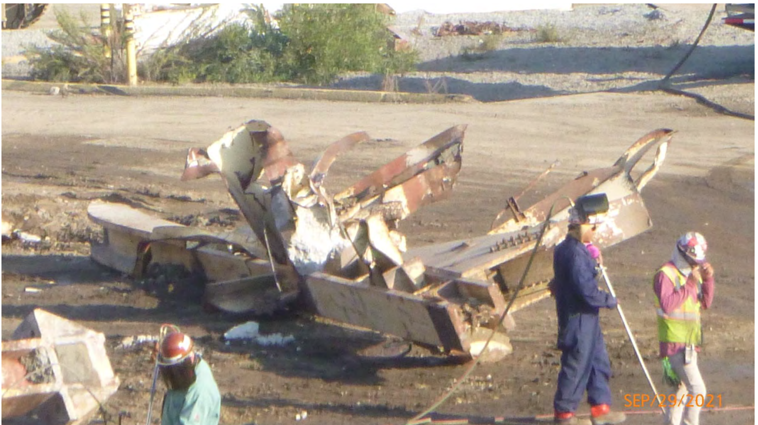
Photo #11: Cutting Structural steel for loading onto trucks lower left fire watch, worker in blue fire suit cutter, worker yellow vest supervisor all with required PPE
