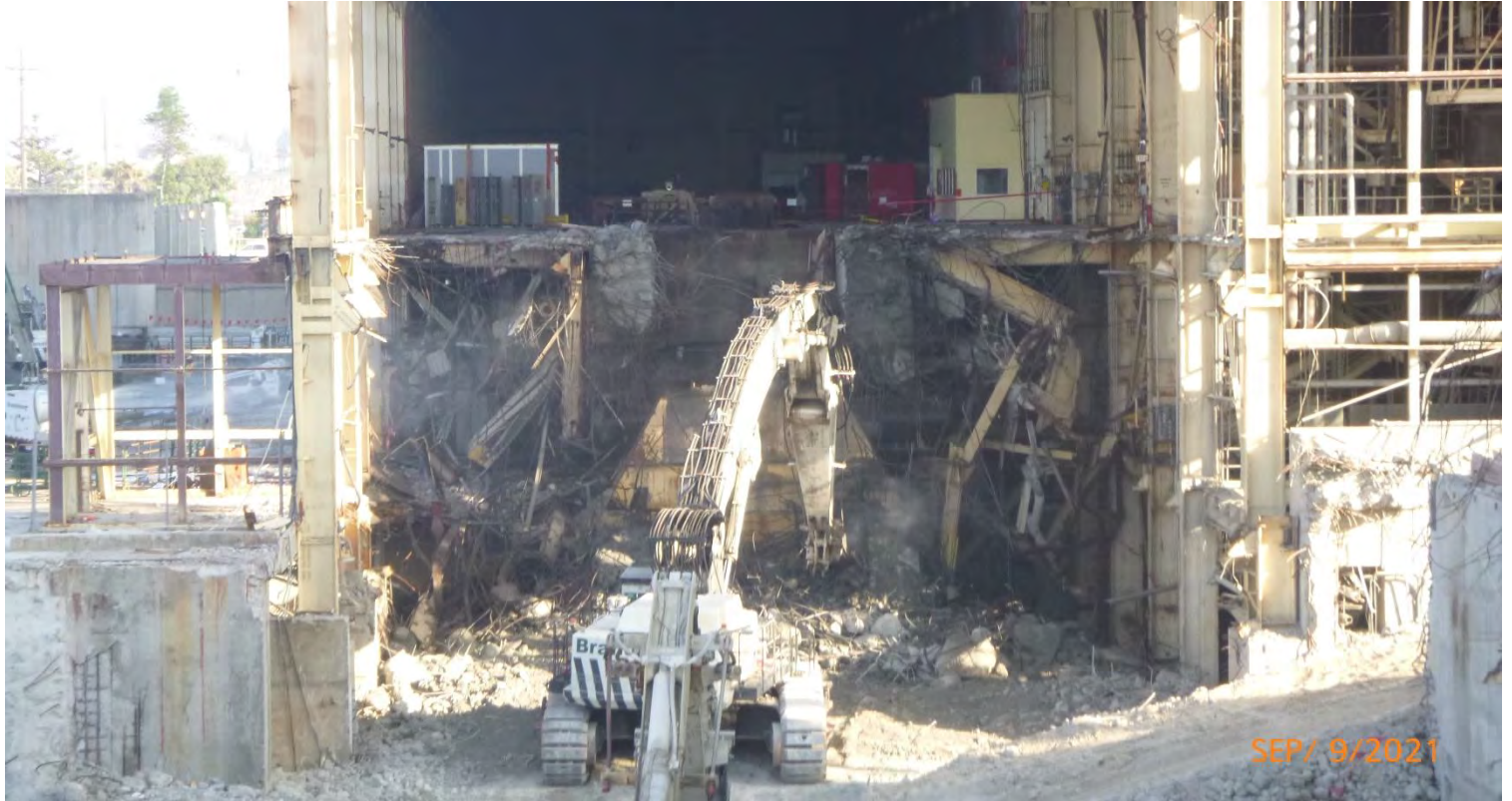
Photo #6: Closeup of Unit #4 turbine Fdn Demo
