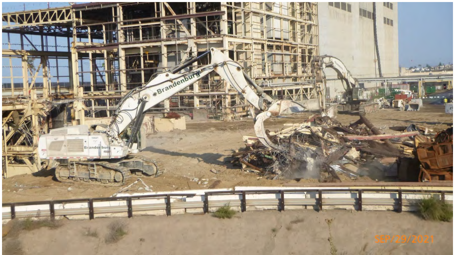
Photo #6: Separating misc. steel for recycle. (b)
