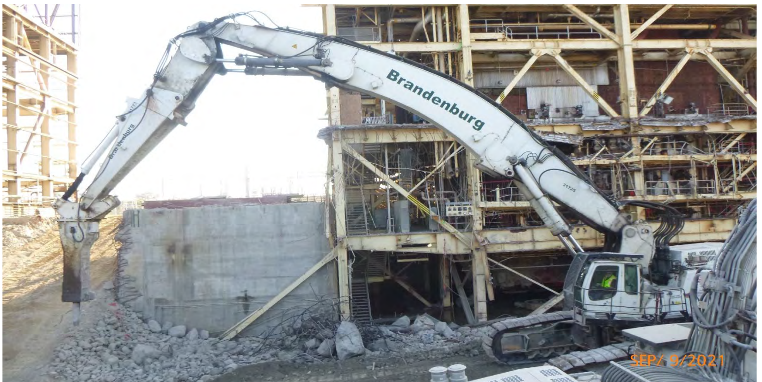
Photo #17: Large Excavator Demo Chipper new to site
