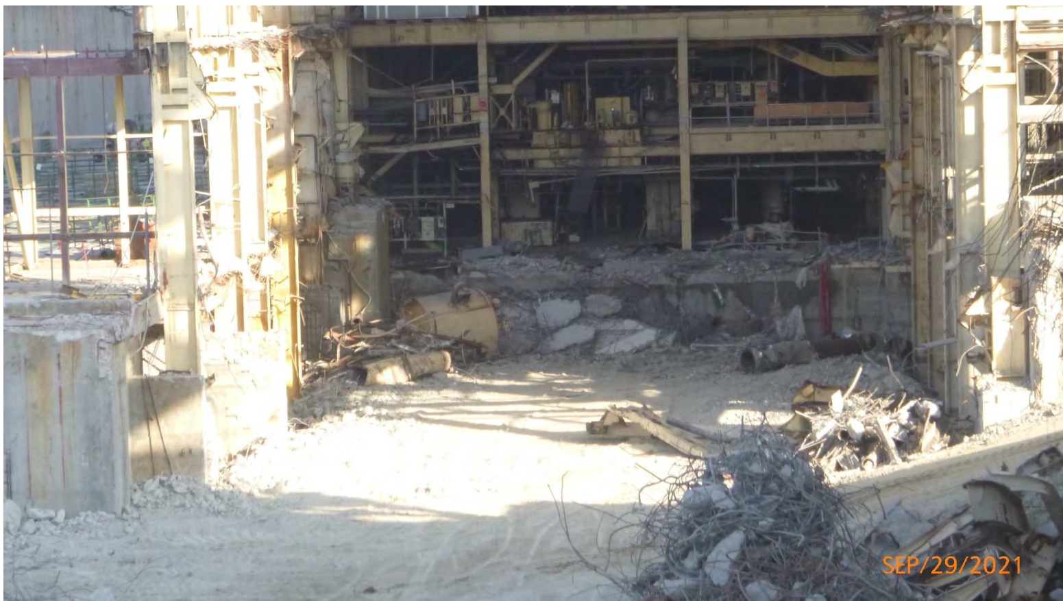
Photo #9: Unit #4 Turbine bay Fdn removed
