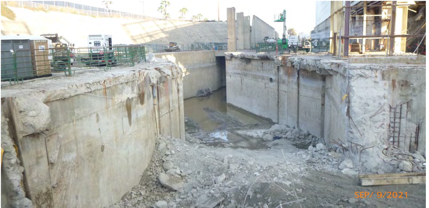
Photo #12: Water Channels in progress to be backfilled
