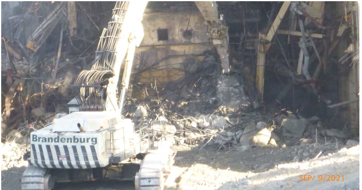
Photo #10: Chipping at Foundation
