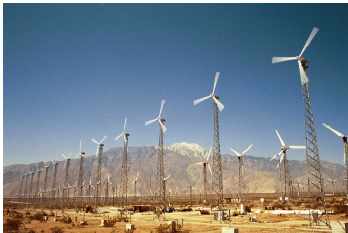
Figure 6. AASI multi-turbine windplant in Palm Springs, CA, which will be used for field test of the integrated wind-to-H 2 system to guide system design improvement. This is the ideal test bed for this project: high-energy wind regime, off-shelf 50 kW nameplate squirrel cage induction motors as generators, simple turbine controls, accessible site, easy scale-up of experimental results to multi-turbine and multi-MW windplants, with windplant owned and maintained by applicant. These 13 turbines have operated for over 20 years with acceptable availability in the severe San Gorgonio Pass wind regime, and are in serviceable condition for this project, which will utilize three of them, at most. In-kind. Windplant operating: https://vimeo.com/86851009
