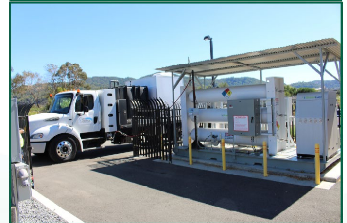
Time-fill RNG Station ( top picture ) and Fast-fill CNG station ( bottom picture ). (Credit: Las Gallinas Valley Sanitary District)
