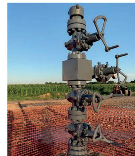
Left: Capped sequestration well. In the industry this set of valves on the well is called the ‘Christmas Tree.’ This well will be used as a monitoring well once the actual CCS well is operational
