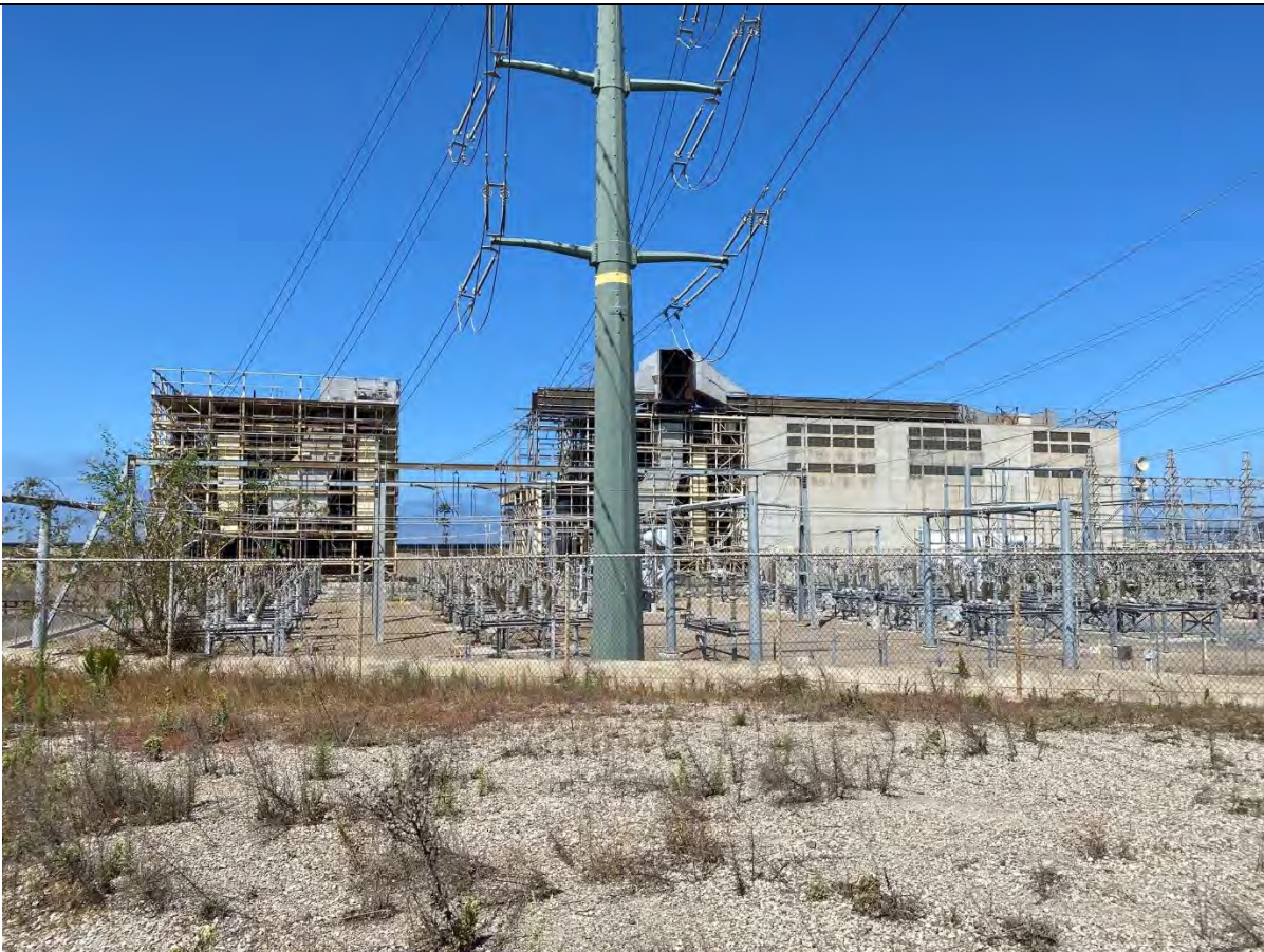
Photo #4: Image of the east side of the project looking west. From this angle it can be seen that Unit 5 (to the left) is now completely separated from the remaining portion of the building.
