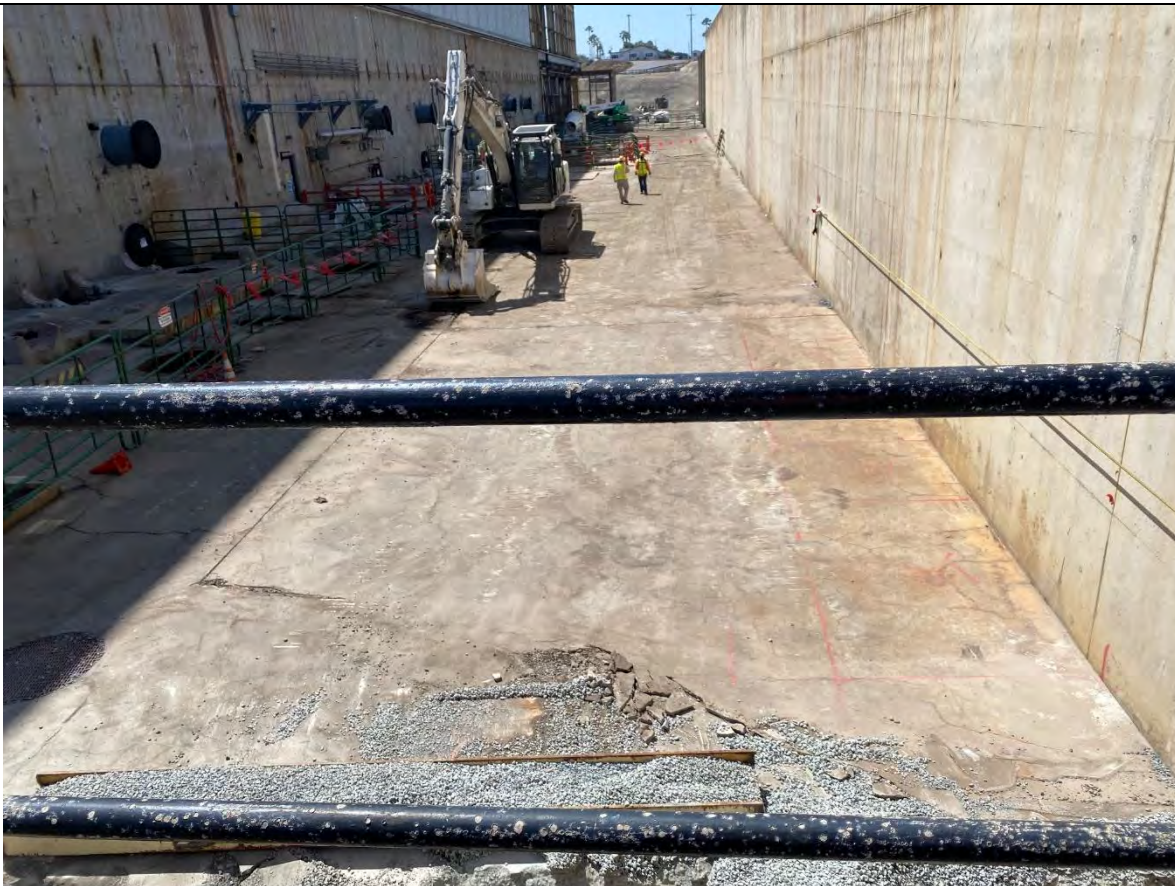
Photo #10: Here is a view of the tunnel lid. Holes will be punctured in the lid about every 10-feet to allow for the fill material to be placed within the tunnel.
