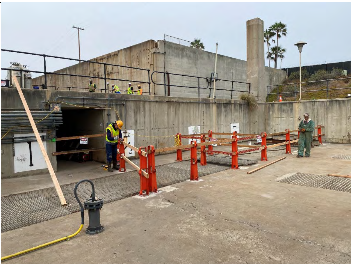
Photo #9: Guards are currently being placed and the grates will then be removed to allow access for the filling of the tunnels.
