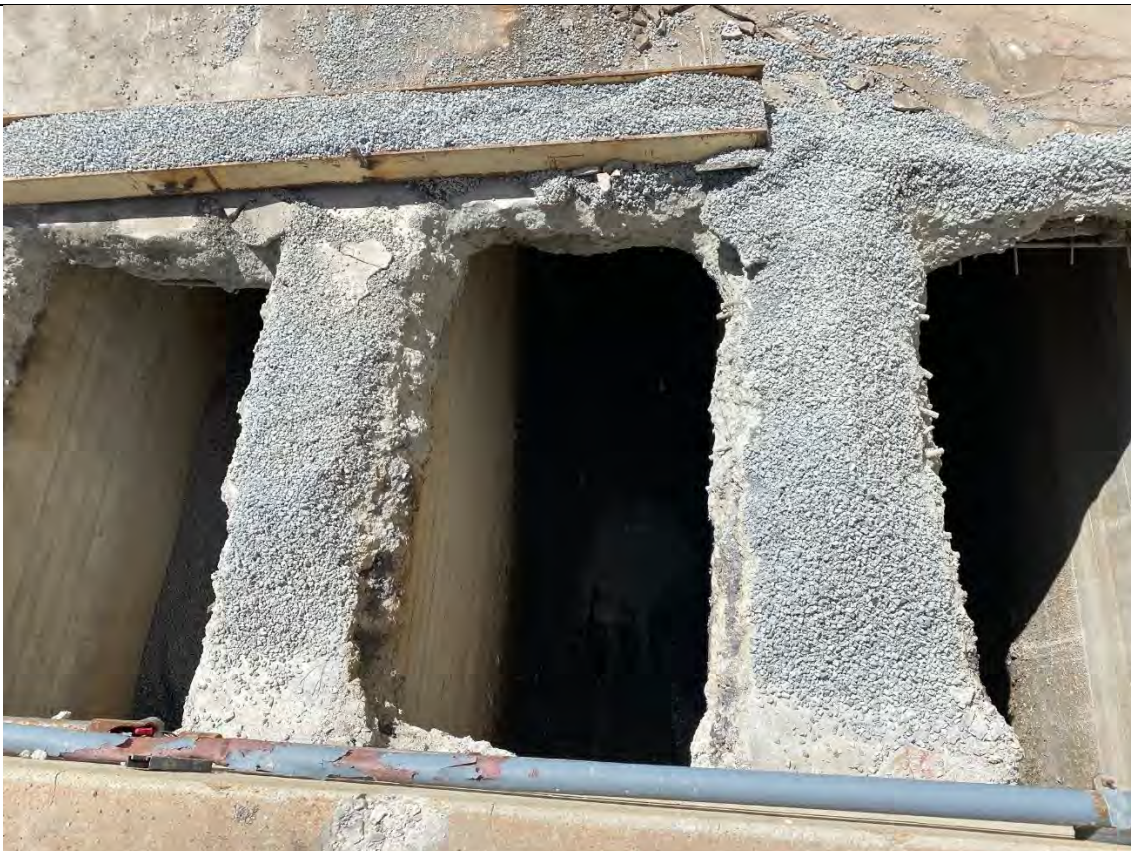
Photo #11: Here is a view of the openings in the tunnel lid and the \frac{3}{4} -inch crushed aggregate that has begun to be placed in the tunnel. The aggregate will be placed to within a foot or two of the lid and then a flowable fill will be placed for the upper portion.
