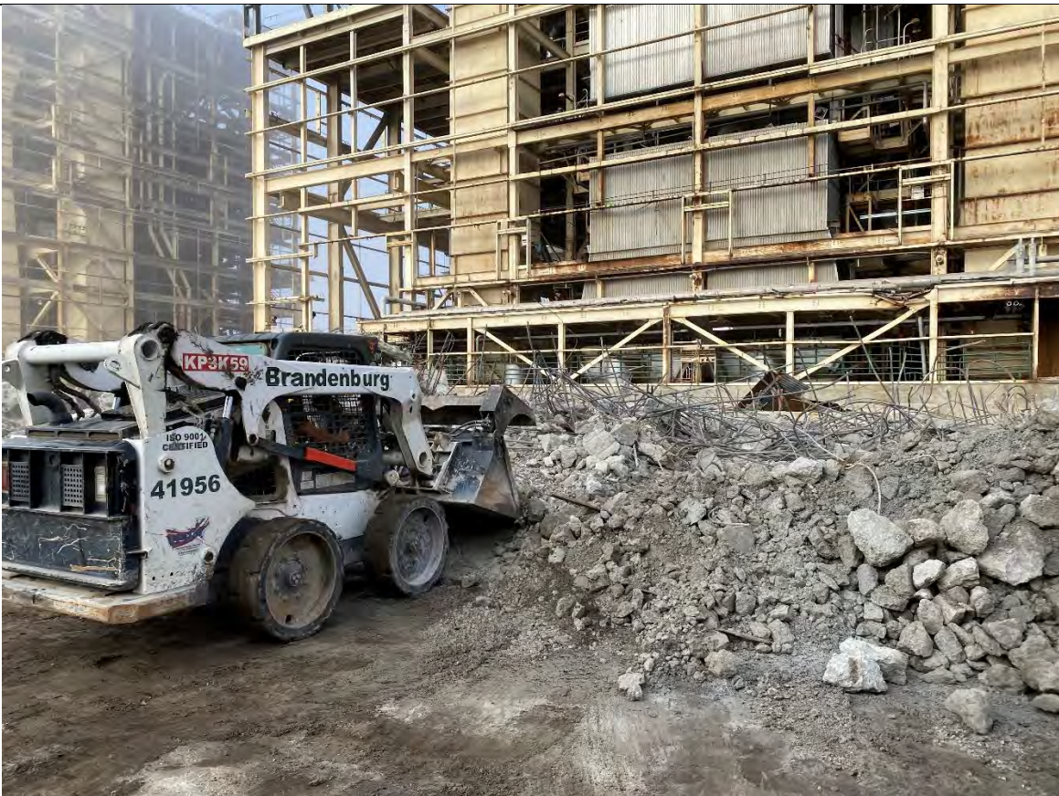
Photo #5: In designated areas debris has been piled and is loaded into dumpsters for removal. Areas around the piles appeared to be relatively clean.
