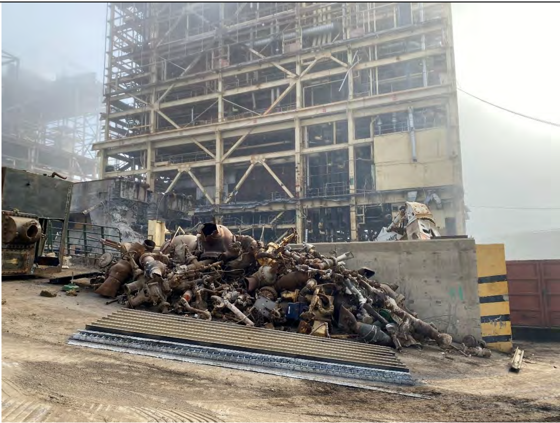
Photo #14: As shown in previous photos, this photo shows stockpiling of specific materials and shows how good housekeeping has been maintained around the piles.
