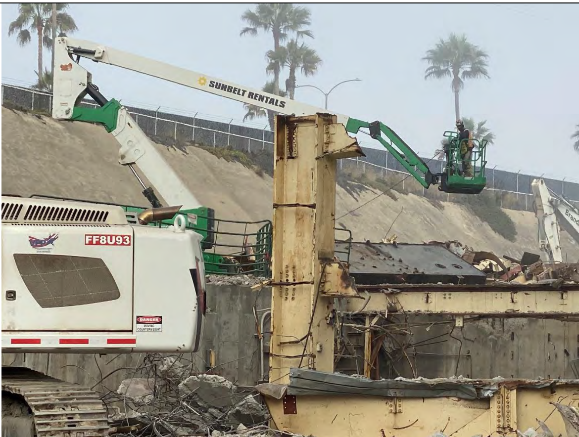
Photo #12: This photo shows a worker in a manlift that cut the larger sections of structural steel and then the larger equipment shown on the left pulls it and places it in the appropriate dumpster or pile.
