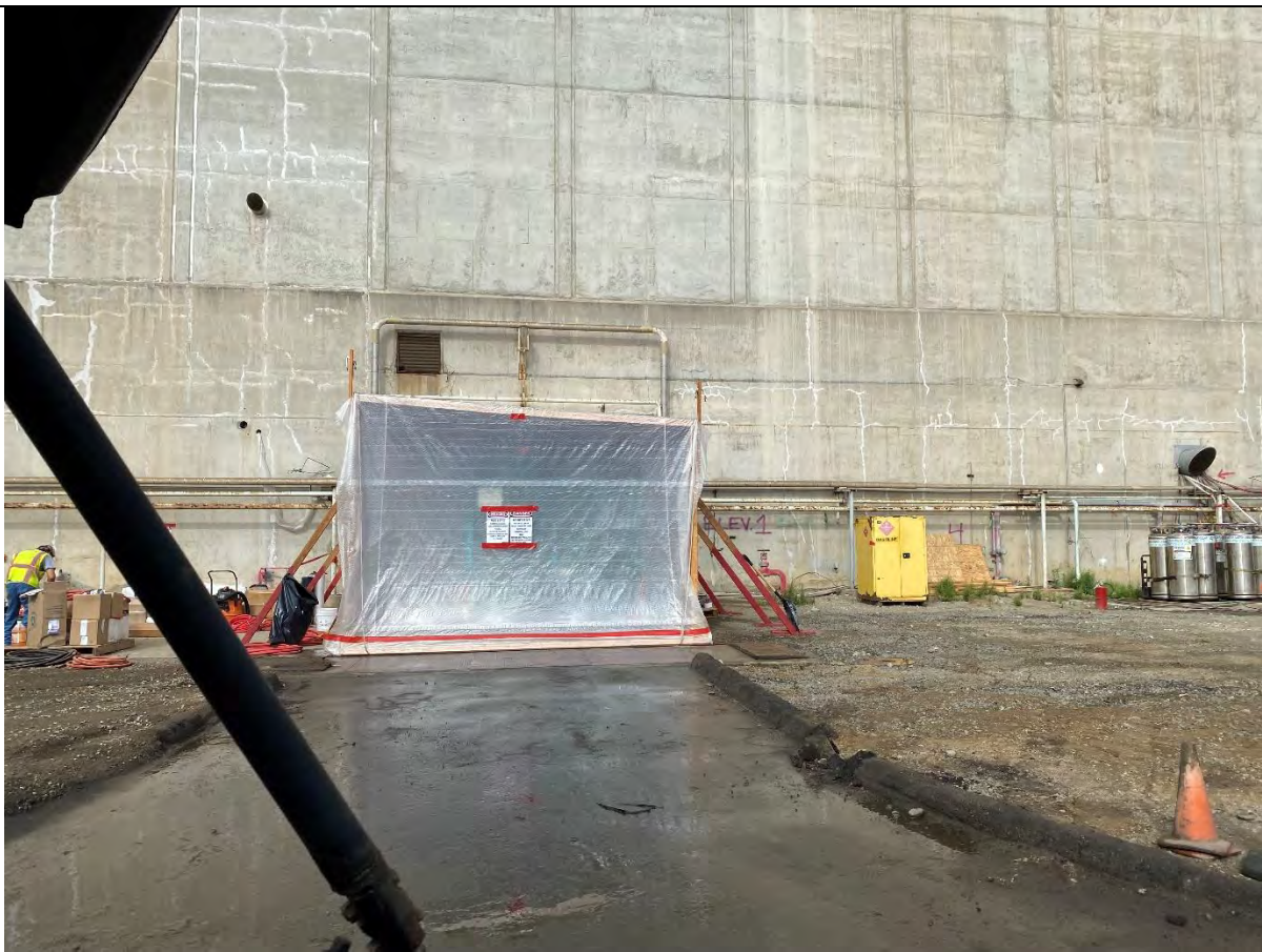
Photo #8: This is a view of the entrance at Unit 2 where asbestos removal activities are still underway.
