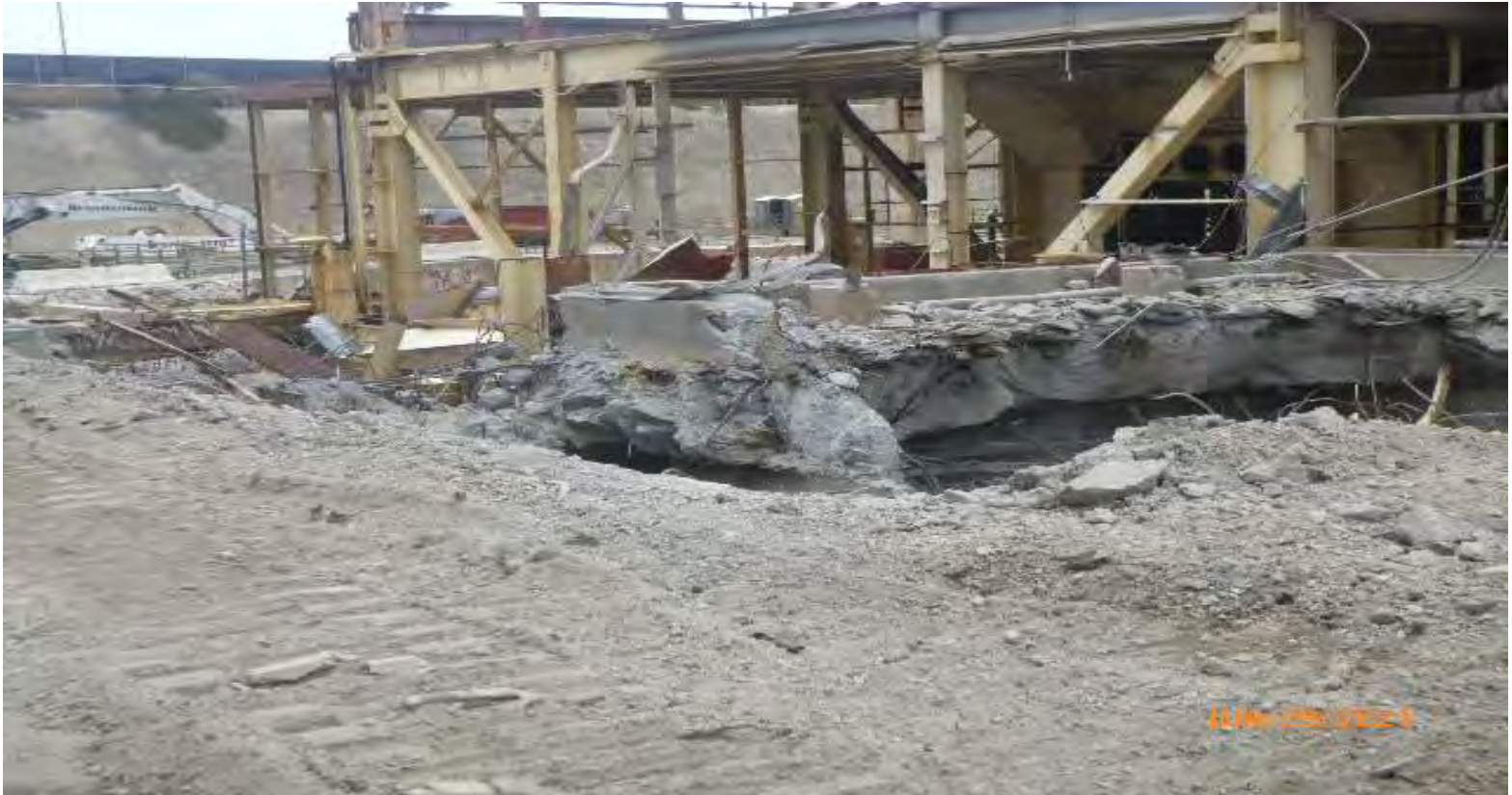
Photo #2: Slab thickness at floor levels typical
