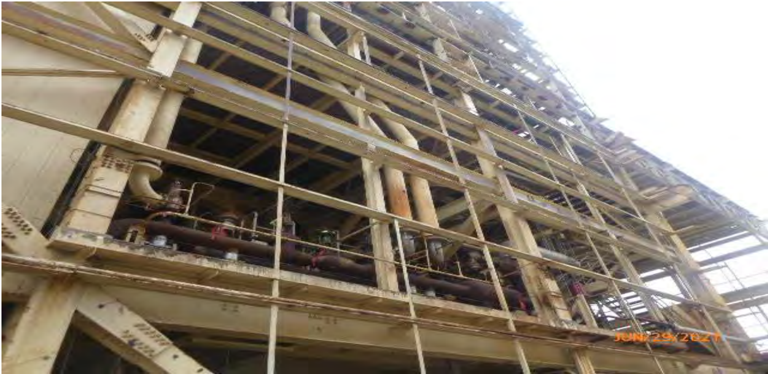
Photo #3: Vertical face after Transite Panel Removal
