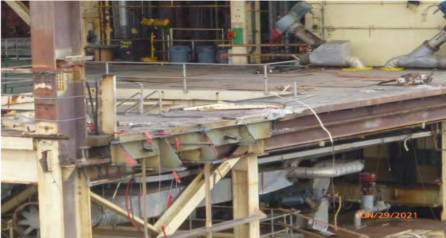
Photo #10: Point of attachment of Rail Bridge (removed)
