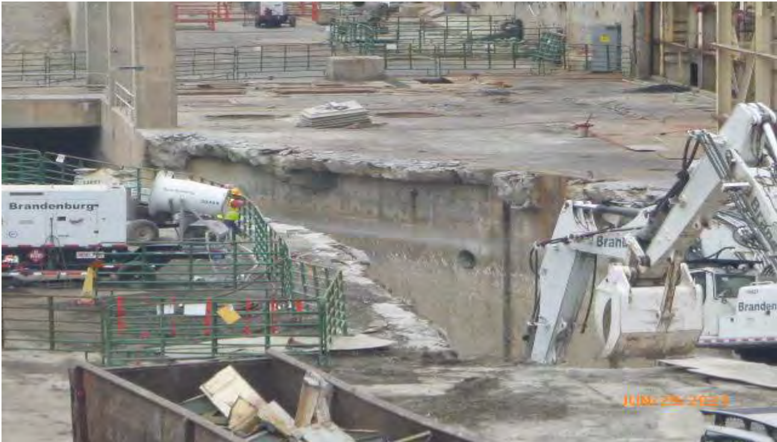
Photo #18: Excavator working on ramp to water channels.
