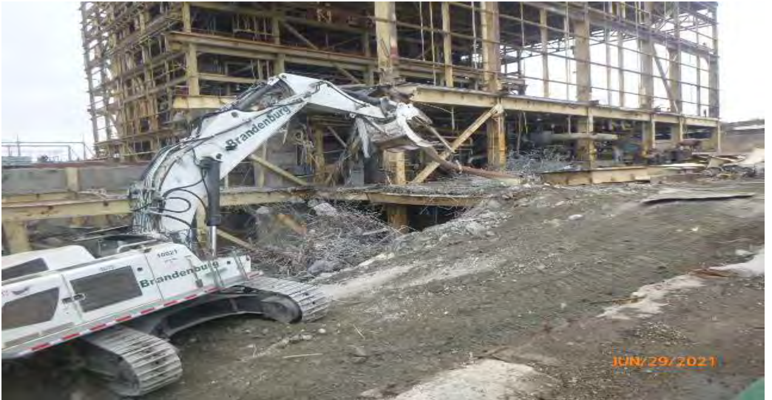
Photo #16: Clearing debris from ramp.
