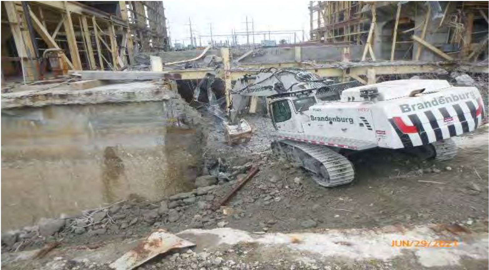
Photo #15: Constructing ramp to lower level.
