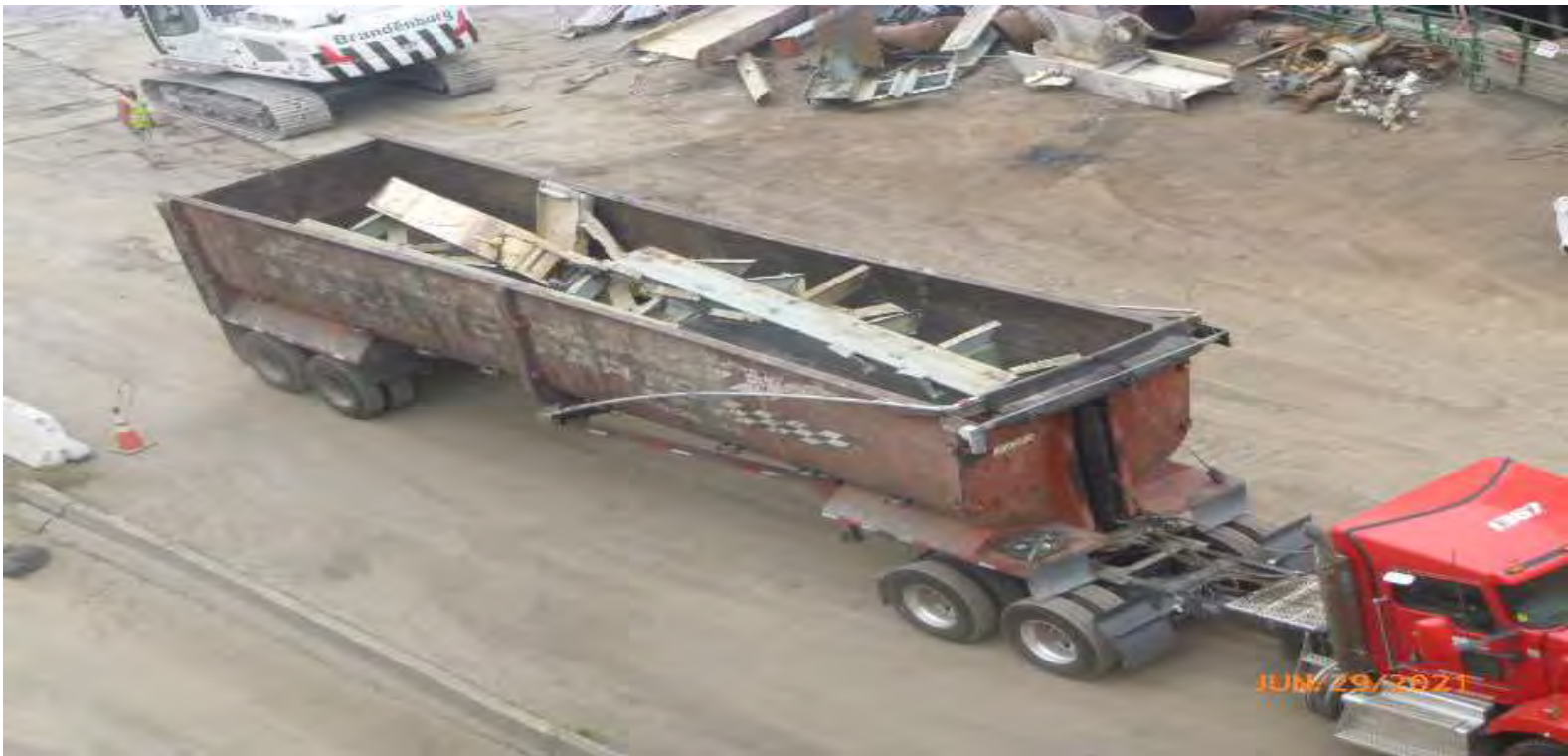
Photo #9: Loaded truck leaving site.
