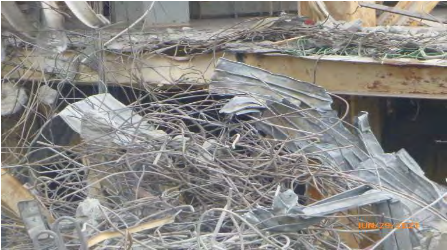
Photo #17: Rebar Pile awaiting haul away.
