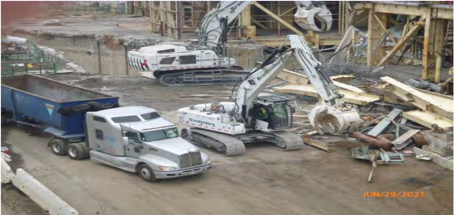
Photo #12: Excavator with claw separating steel prior to loading
