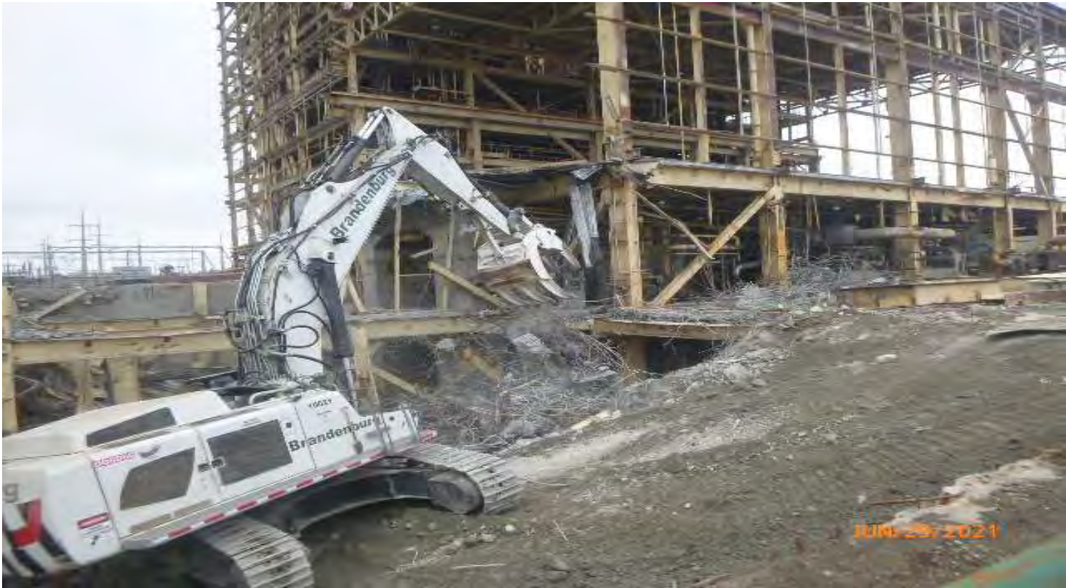
Photo #14: Excavator separating rebar.
