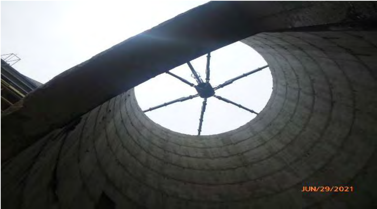
Photo #5: View vertical inside remaining stack.
