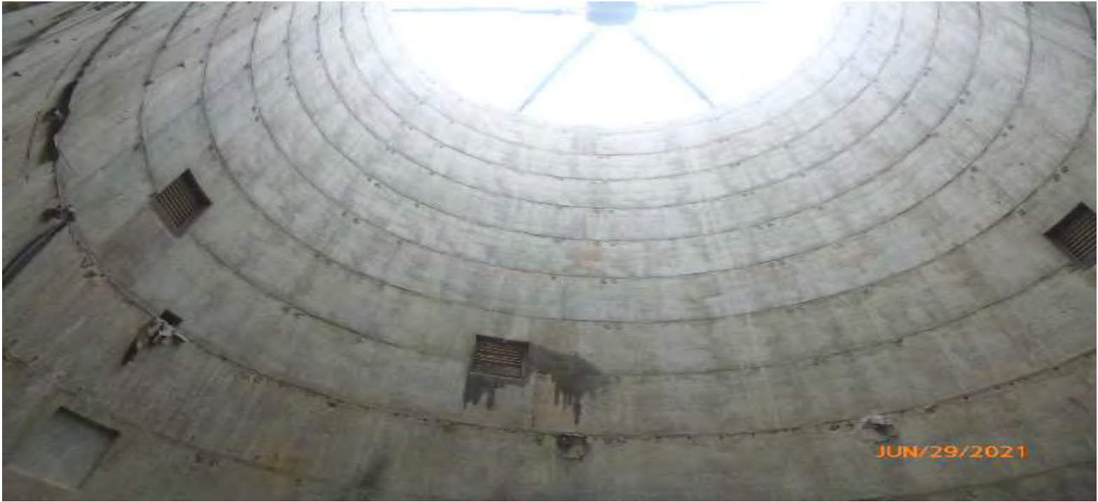
Photo #6: Inside Stack walls
