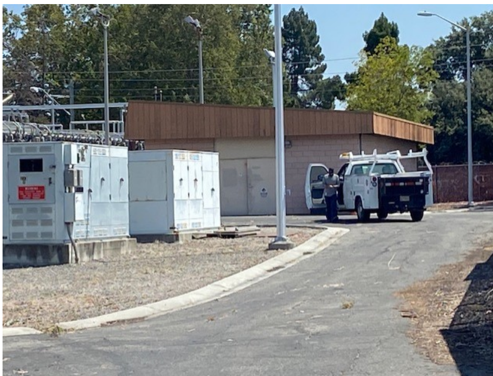
Photograph 2. Substation building north elevation; facing south.
