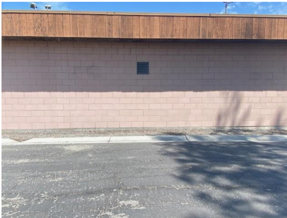
Photograph 3. Substation building west elevation; facing east.
