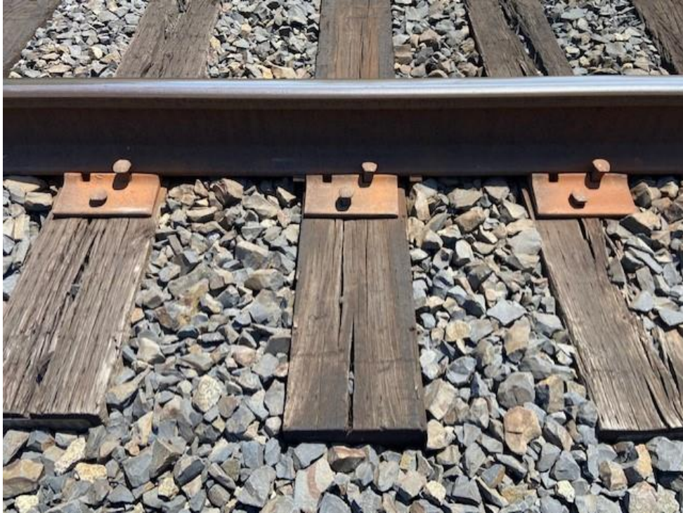
Photograph 3. Detail of track materials and construction.
