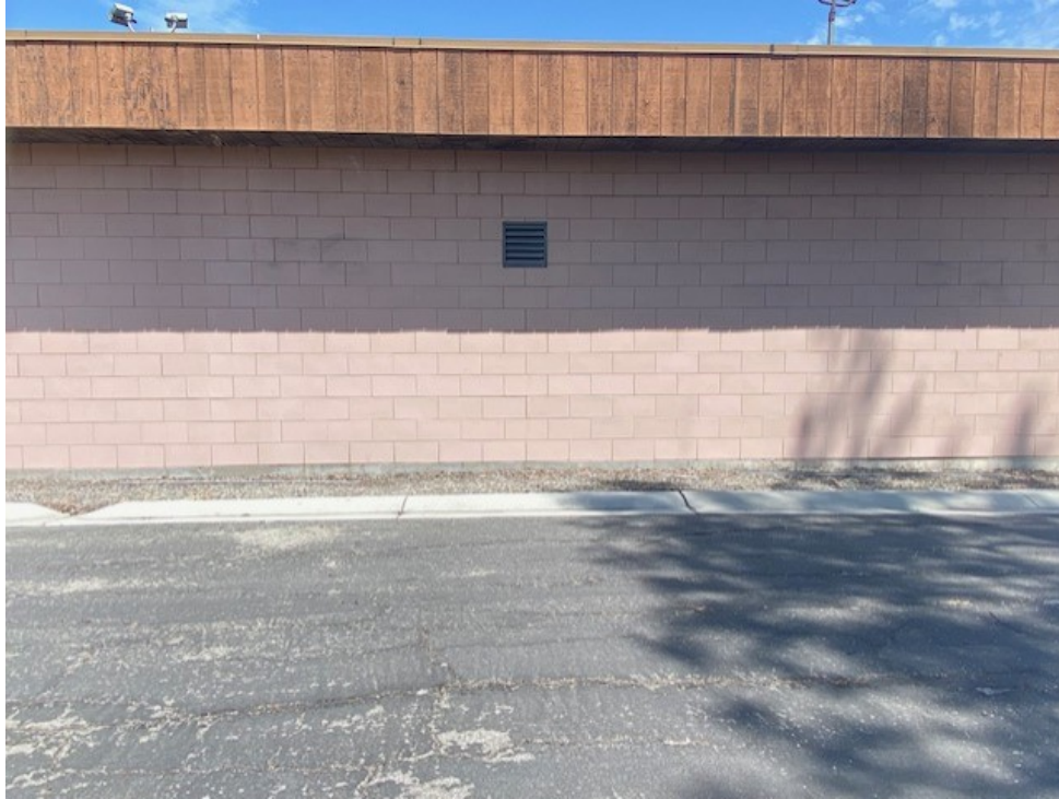
Photograph 3. Substation building west elevation; facing east.
