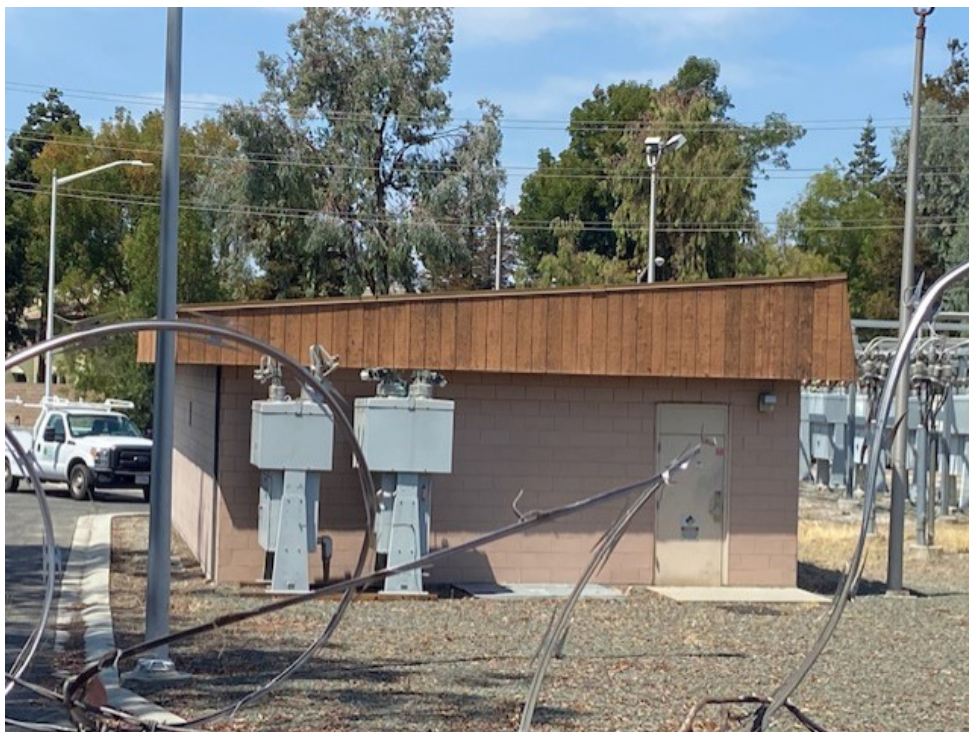
Photograph 4. Substation building south elevation; facing north.
