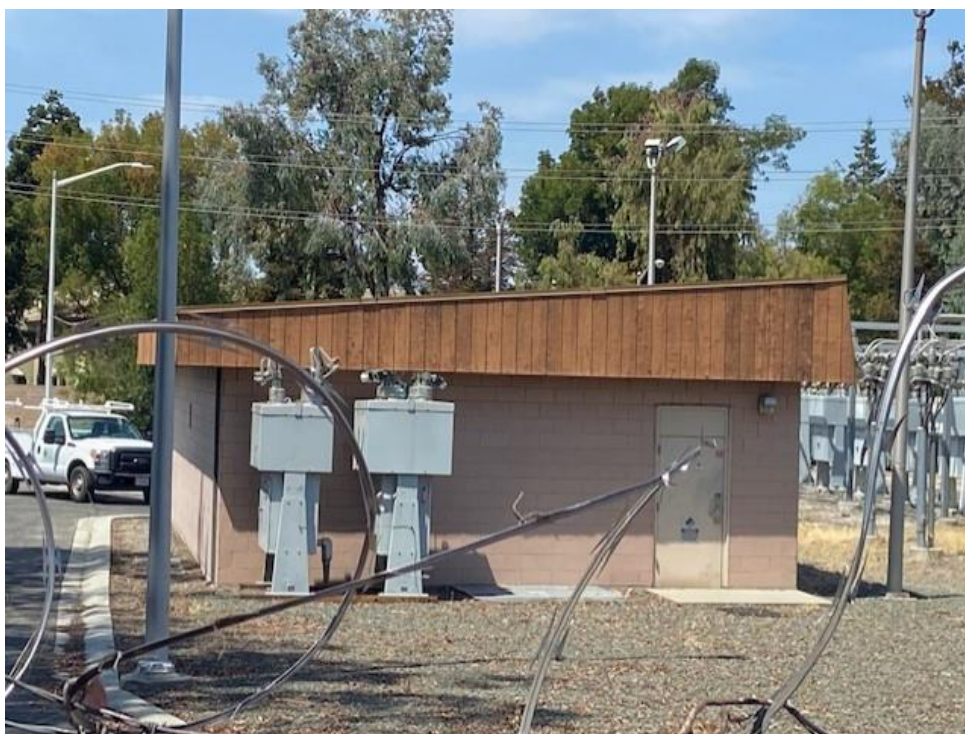
Photograph 4. Substation building south elevation; facing north.
