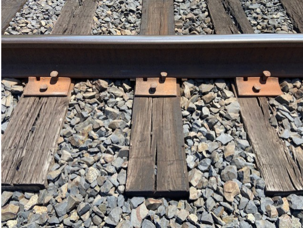
Photograph 3. Detail of track materials and construction.
