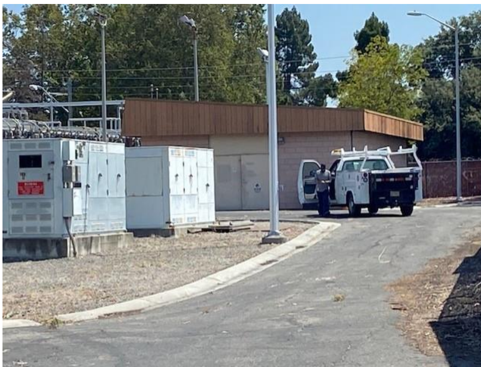
Photograph 2. Substation building north elevation; facing south.
