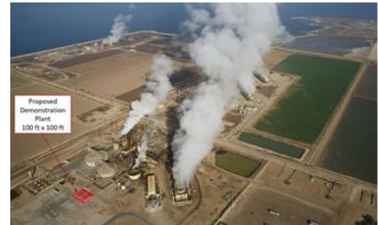
The demonstration system at a geothermal power plant in Calipatria, California
