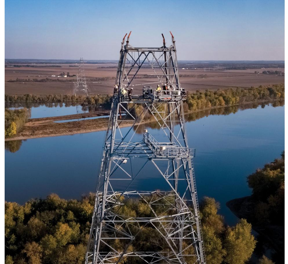
Construction of a lattice tower structure crossing the Illinois River; part of the Illinois Rivers Transmission Project
