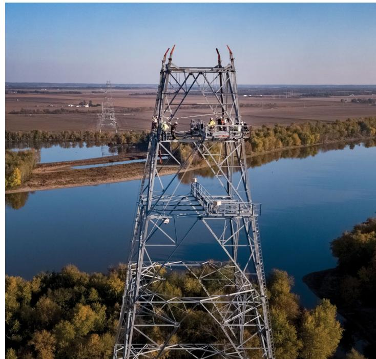
Construction of a lattice tower structure crossing the Illinois River; part of the Illinois Rivers Transmission Project
