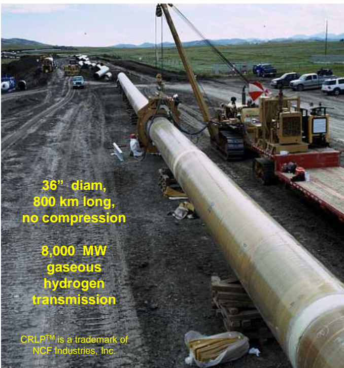
Hydrogen Embrittlement resistant option: Composite Reinforced Line Pipe (CRLP) FRP (fiberglass) hoop strength over mild steel core
