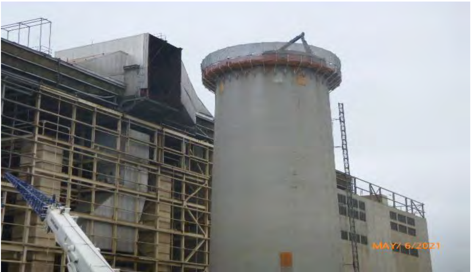
Photo #1: Stack demo halted due to equipment breakdown. Remaining 138'.
