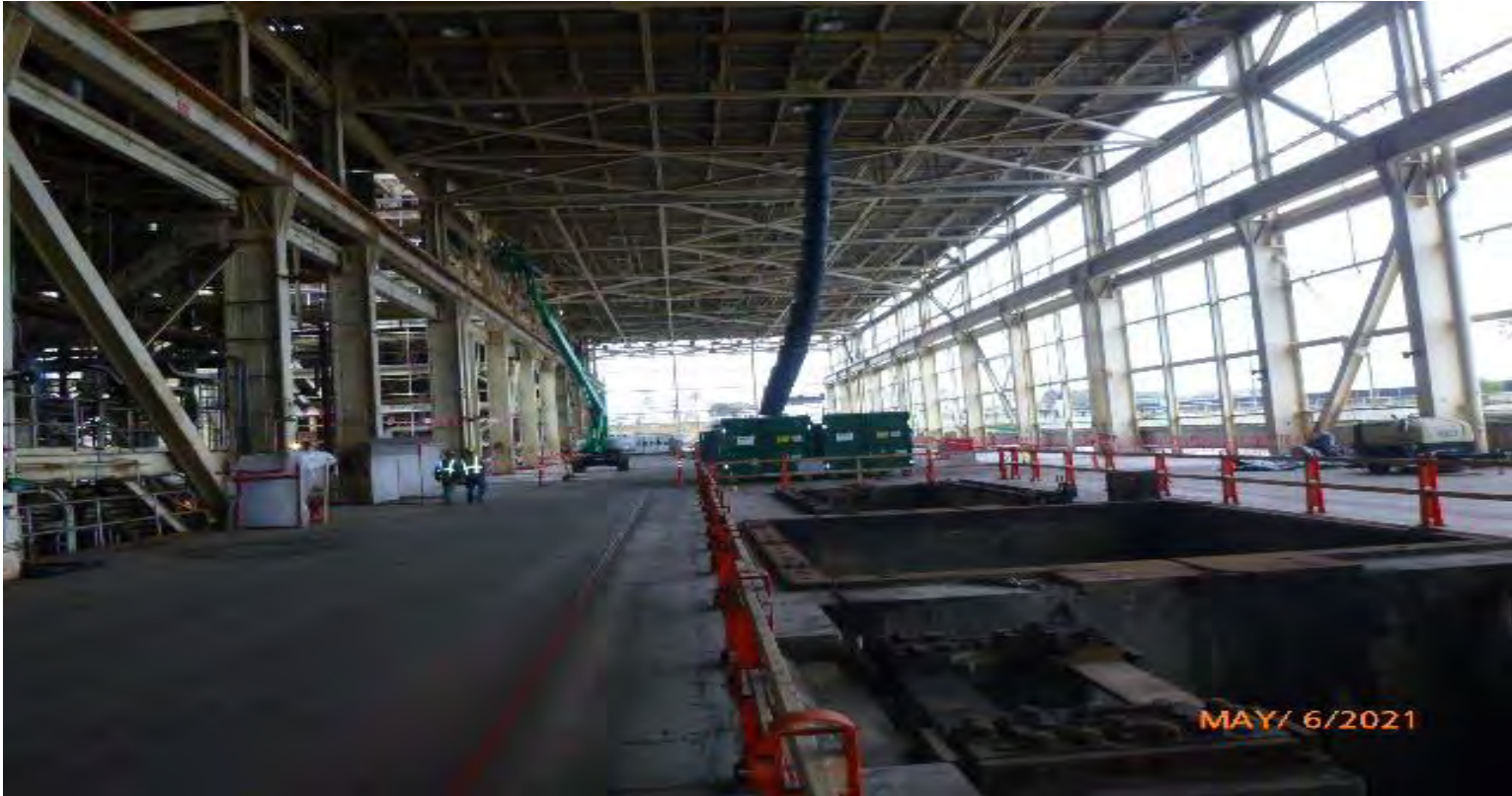
Photo #6: Roofing Demo in progress at roof of Turbine Building
