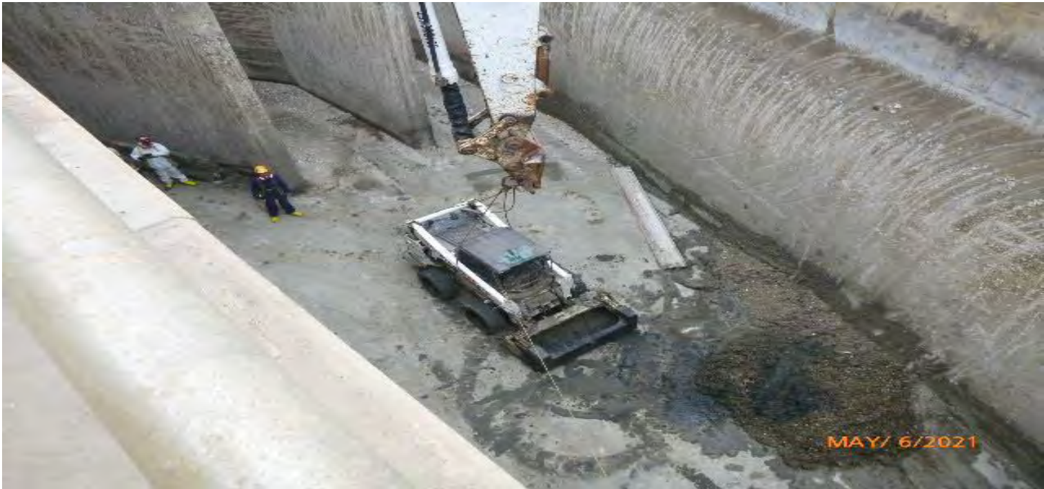
Photo #7: Sequence photos of lift of skid loader from water channel below (1)
