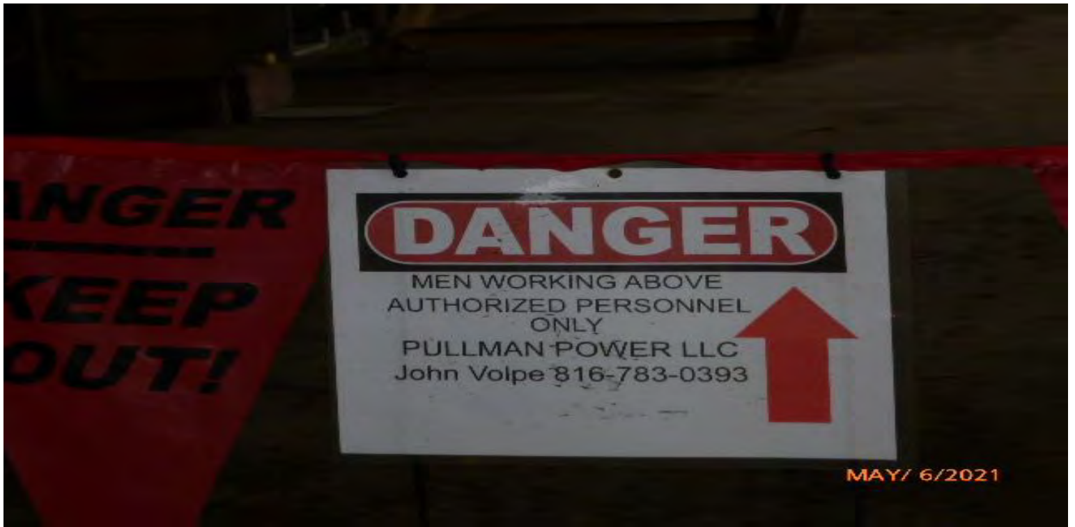
Photo #4: Signage installed at Stack Demo warning of overhead hazards
