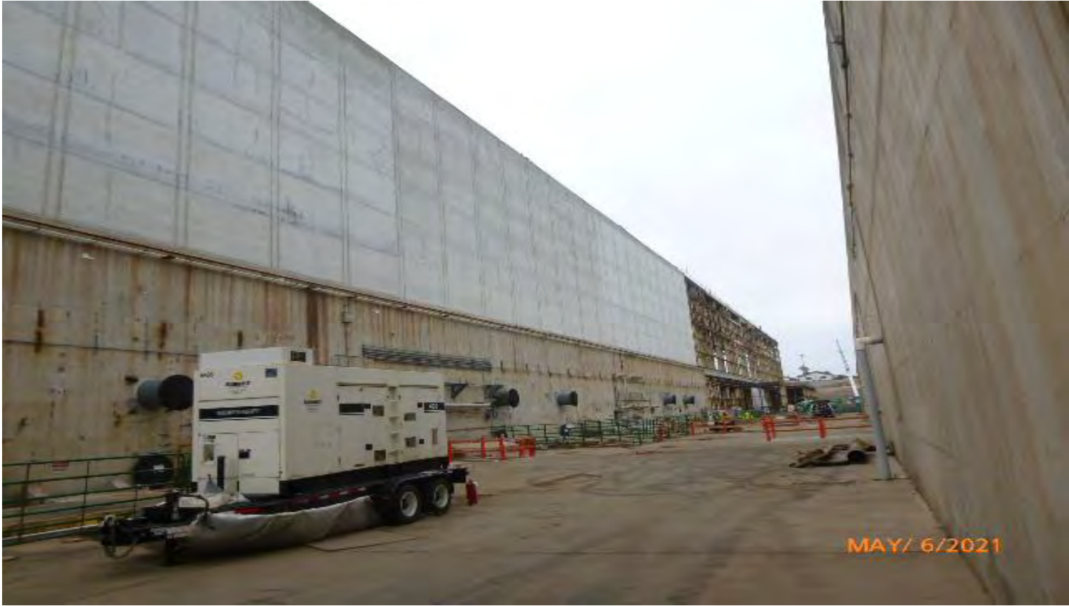
Photo #12: Transite panels removed at west wall clean up in progress
