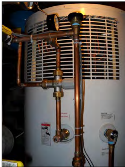
Figure 14. Heat pump water heater with mixing valve
