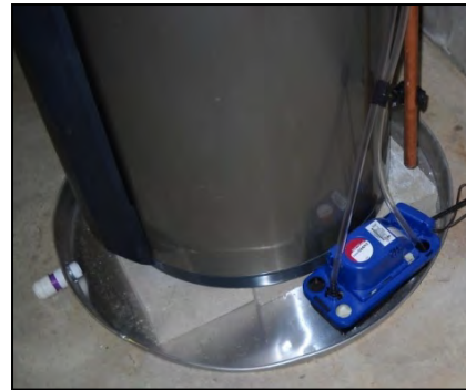
Figure 11. Proper HPWH installation
