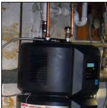
Figure 12. HPWH without heat traps
