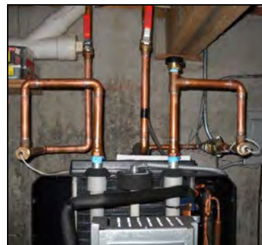
Figure 13. HPWH with heat traps
