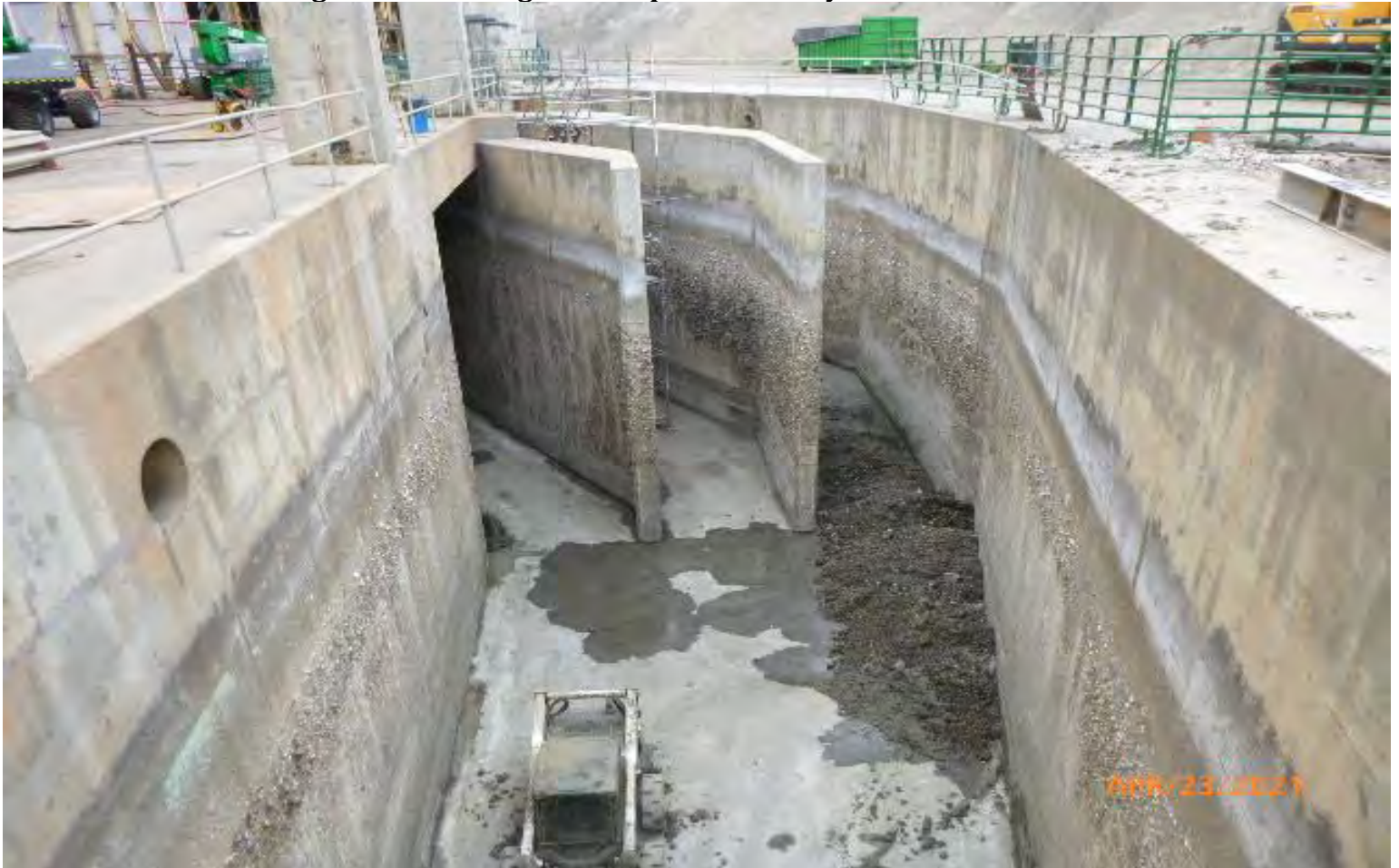
Photo #1: Water Cooling channels being cleaned prior to slurry backfill
