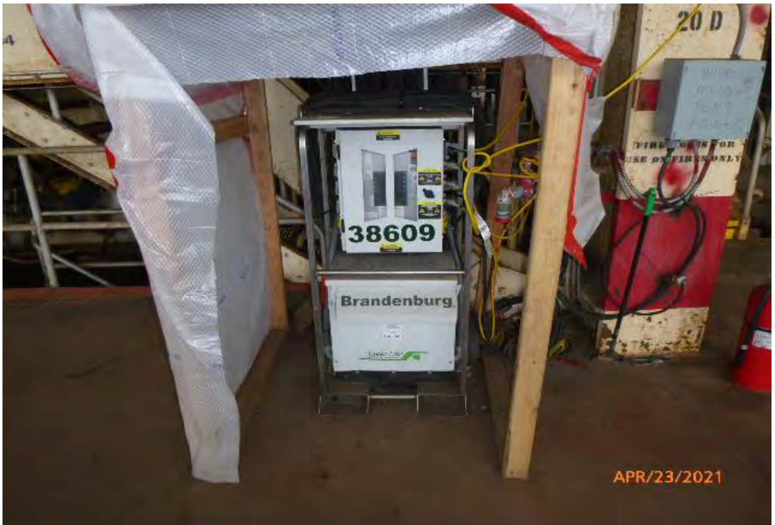
Photo #3: Typical Temporary Power Distribution Unit note extension cords used extensively
