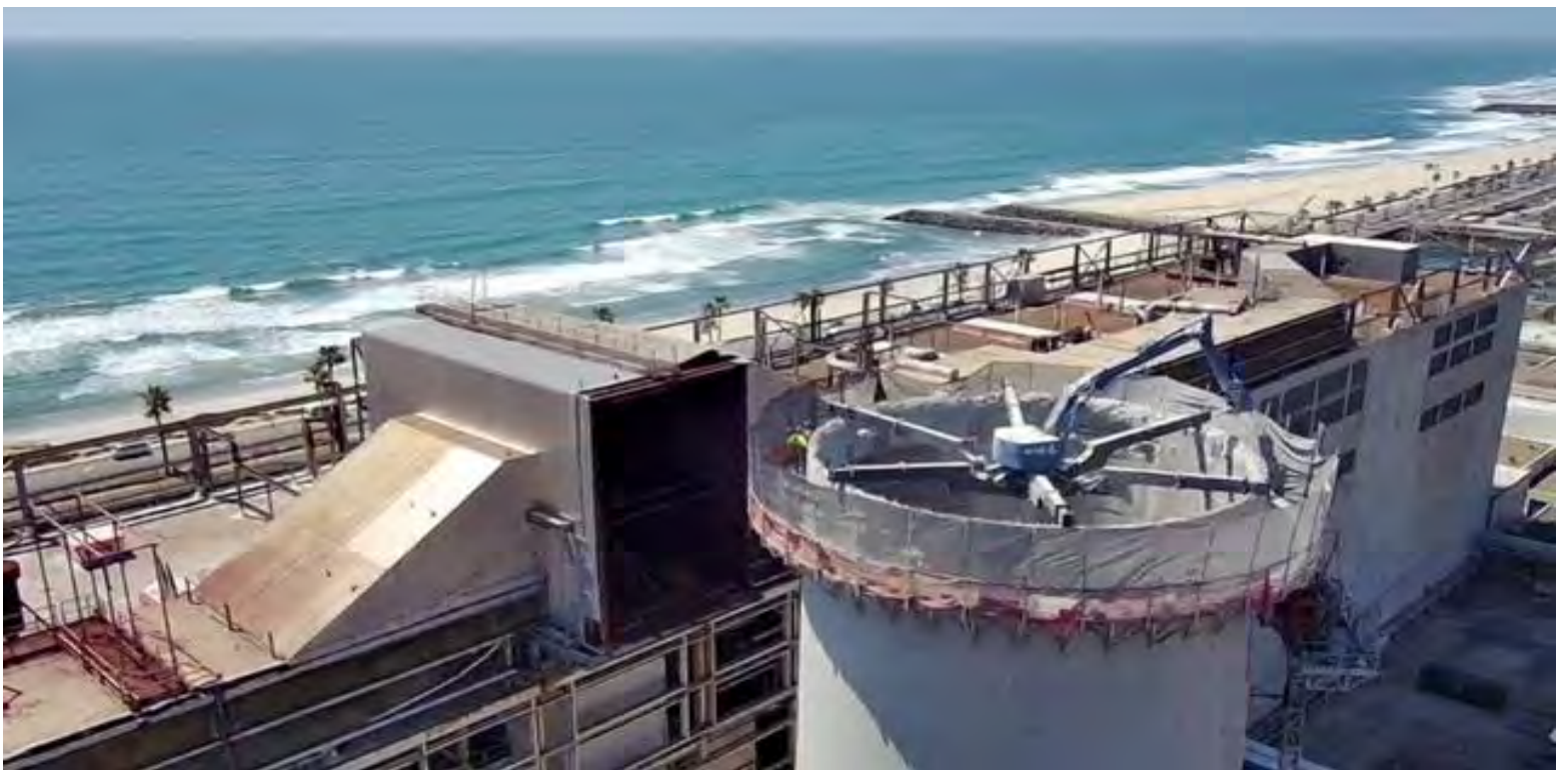
Photo #11: Pullman's Spider at top of stack demo in progress
