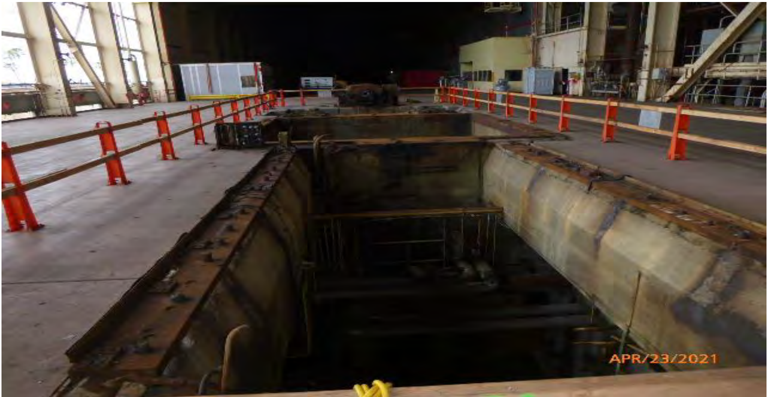
Photo #4: Turbine Removed typical #1 - #5
