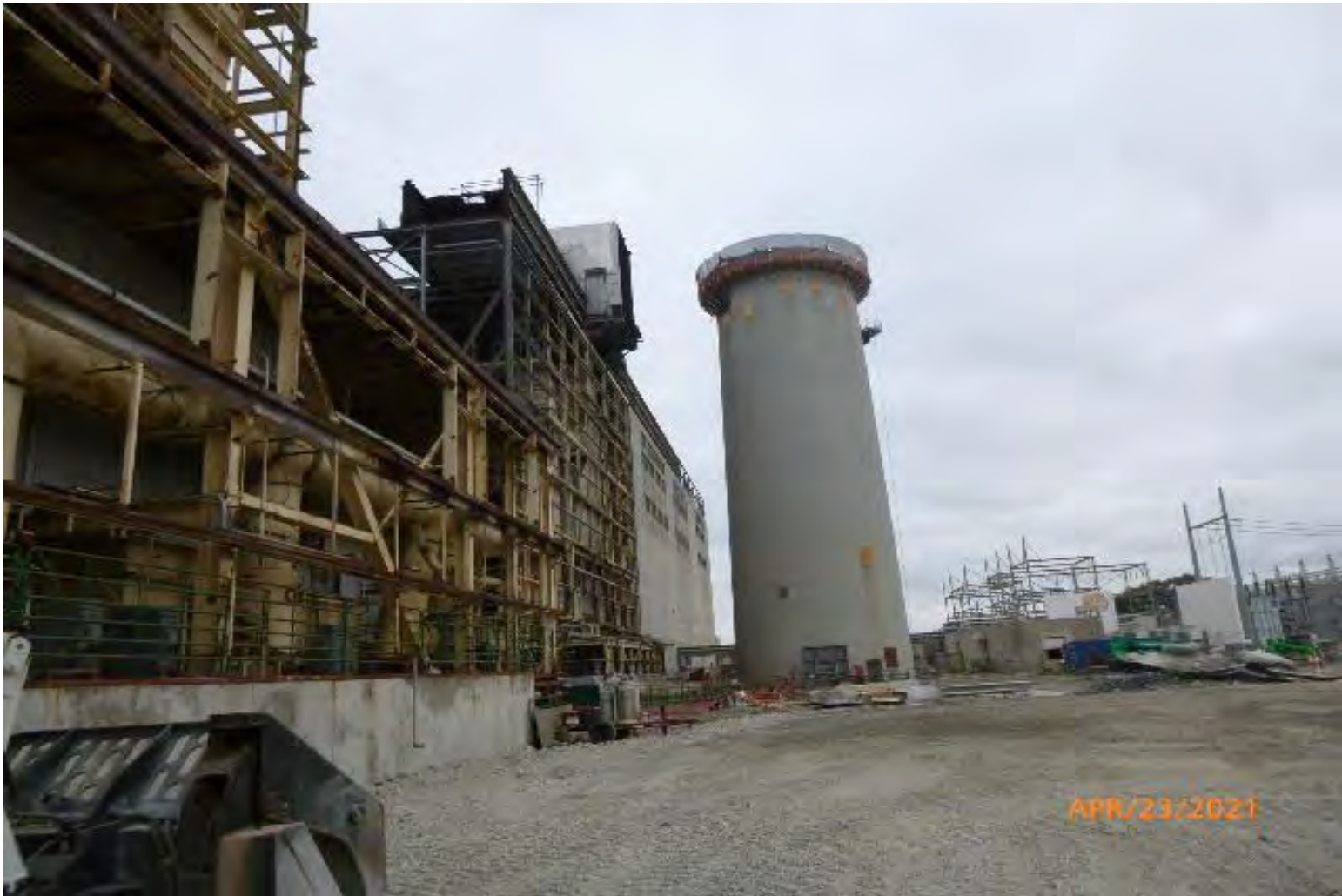
Photo #2: Stack Demo at this time down to approx. 250'
