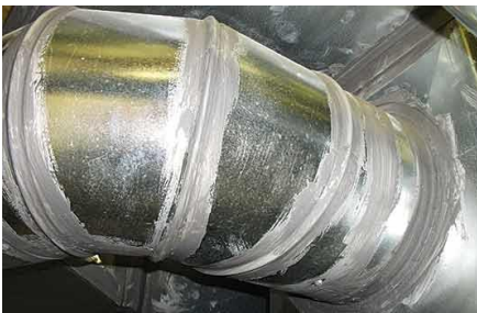
Figure 21: Duct with mastic applied.
