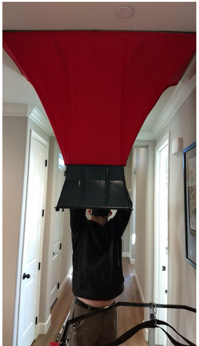
Figure 7: Testing airflow using a non-powered Shortridge flow hood.
