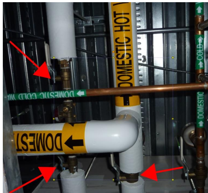
Figure 9: Uninsulated valves.
