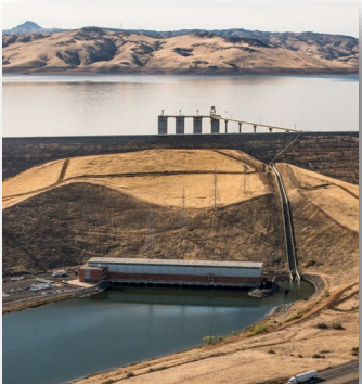
Gianelli Pumping-Generating Plant
