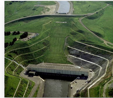
Banks Pumping Plant
